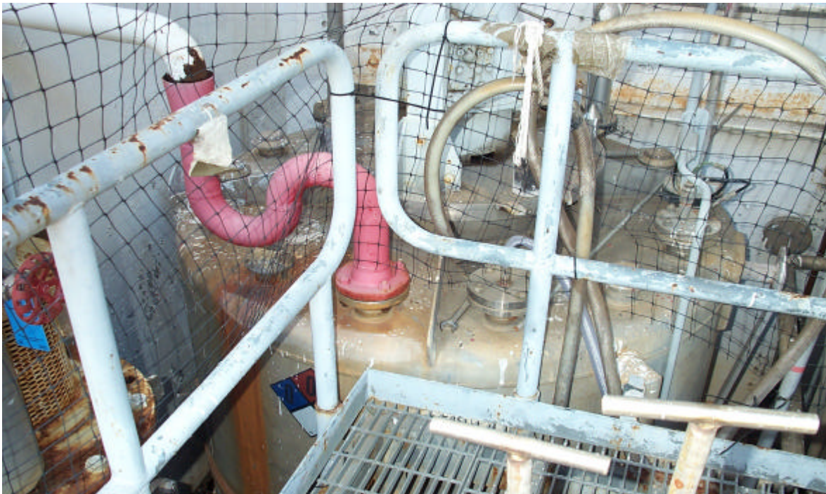
Figure 2-6: Overheads Tank
