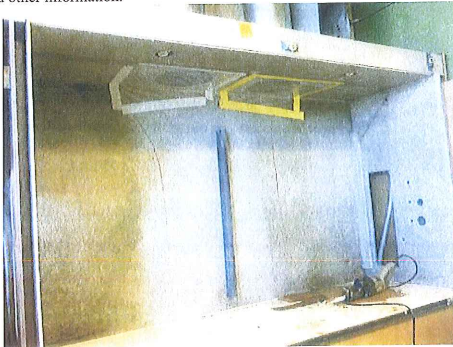
Figure 8. A typical fume hood with steel casing and glass sash removed showing the Transite lining. The bright area on the rear wall is where decontamination was performed. The dark curved lines running from top to bottom indicate the boundaries of the contamination.
