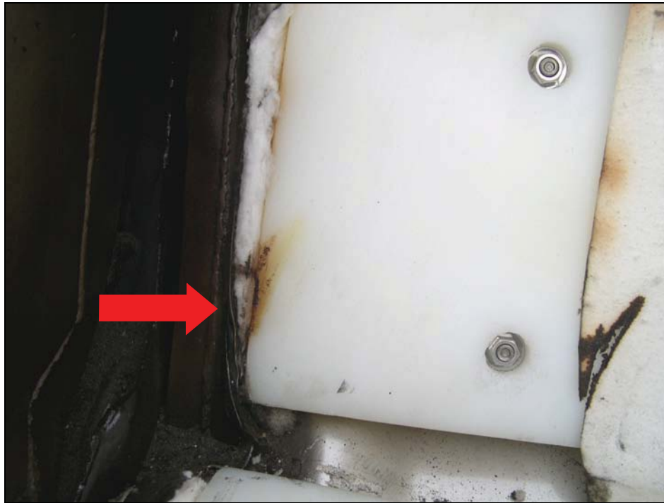
Figure 3-43 Location of Possible Combustion of Moderator
