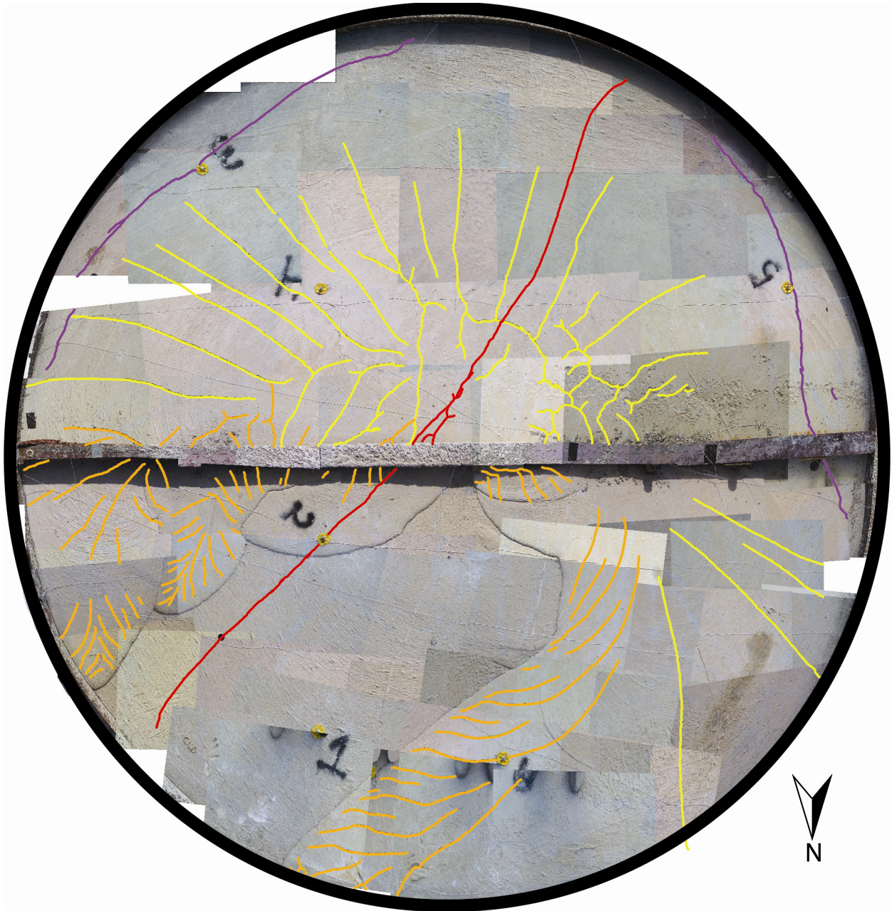
Figure 4-2. Photomosaic of the 6.1-m [20-ft]-Diameter Intermediate-Scale Grout Monolith With Crack Distribution Patterns Traced and Coreholes 1–6 Shown. Yellow Cracks Belong to the Set That Is Radial to the Monolith, Orange Cracks Belong to the Set That Is Perpendicular to Lobe Flow, Red Cracks Are Two Major En Echelon and Several Related Minor Cracks, and Purple Cracks/Crack Families Developed Late Through Coreholes 3 and 5 Concentric to the Monolith Edge.
