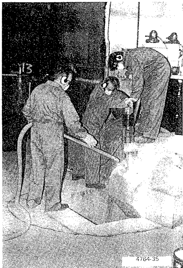
Figure 33. Excavating Concrete From Area Below Primary Reactor Operating Position
