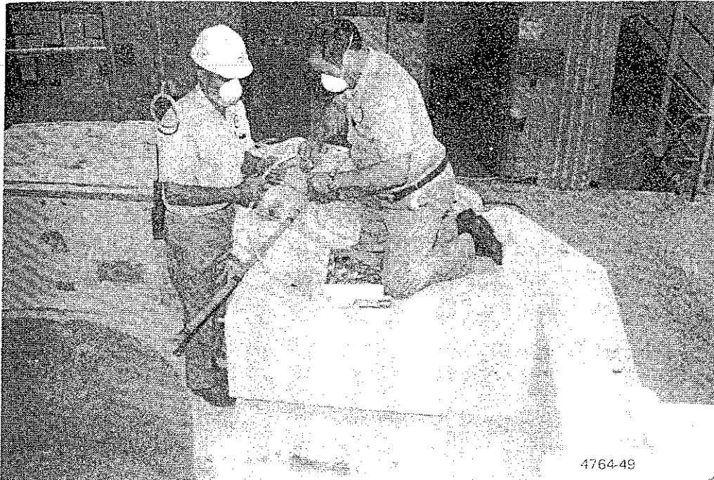
Figure 50. Explosive Charges Being Loaded Into Pre-drilled Holes
