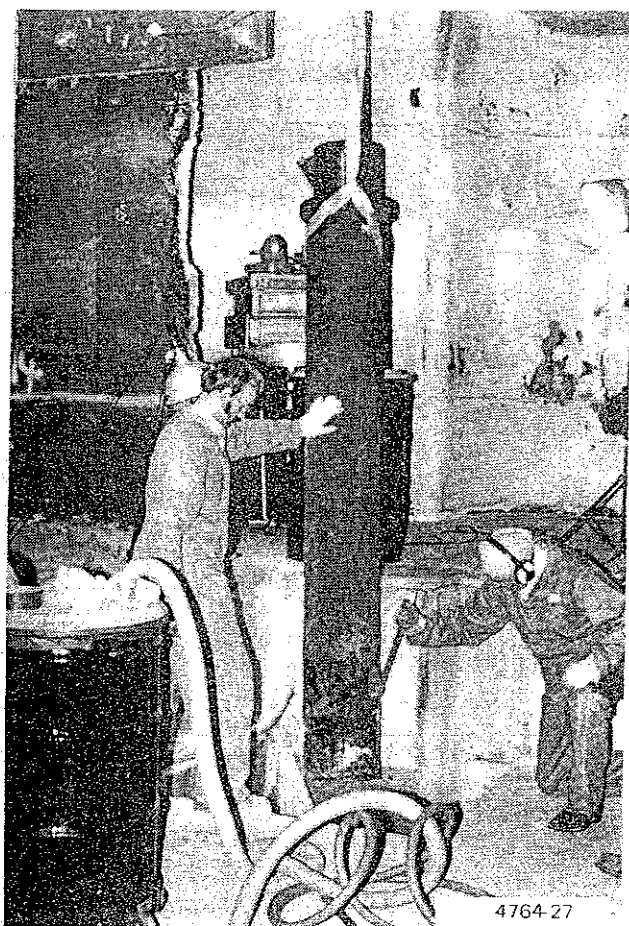
Figure 21. Excavating Sand From Around Lead Shield Hoist
