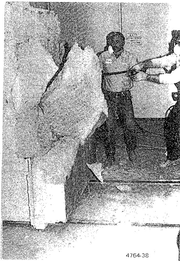
Figure 35. Using a Rock Breaker to Form Cracks in Activated Portion of Rolling Door
