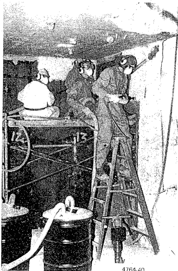
Figure 38. Scabbling Concrete from Surface of Exposure Room Wall
