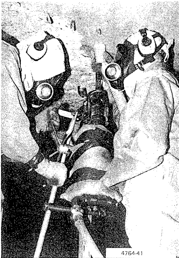
Figure 39. Using Rock Drill to Bore Holes Into Ceiling of Exposure Room (preparation for inserting rock splitter)
