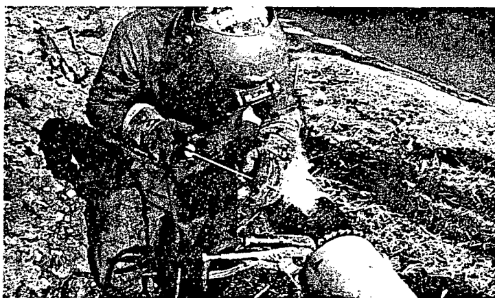
Worker completes a weld in six-inch pipe to be installed in the 10-mile-long Roxbury to Dane natural gas connecting line in western Dane County.
