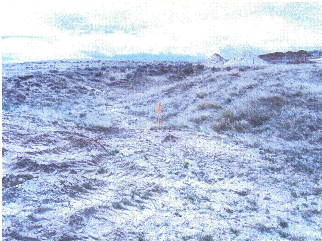
Figure 9b Disturbance in drainage without sediment control
