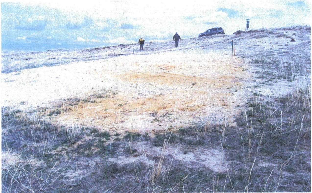
Figure 9a Disturbance area on slope without sediment control
