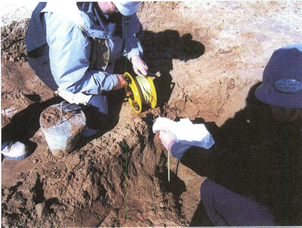
Figure 2 – Measuring depth to plug gel
