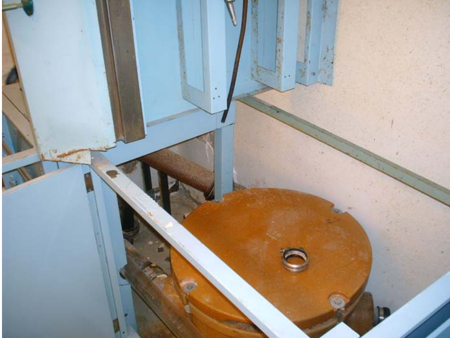
Former Rad Lab (Room 1097) – Removed Piping
