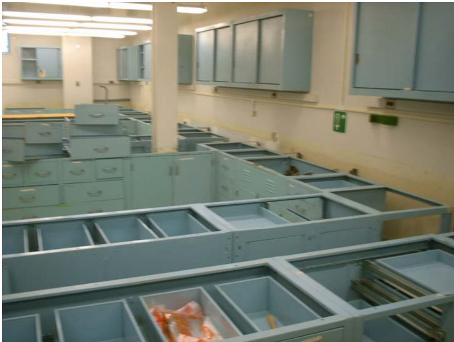
Former Rad Lab (Room 1097) – Removed Countertops
