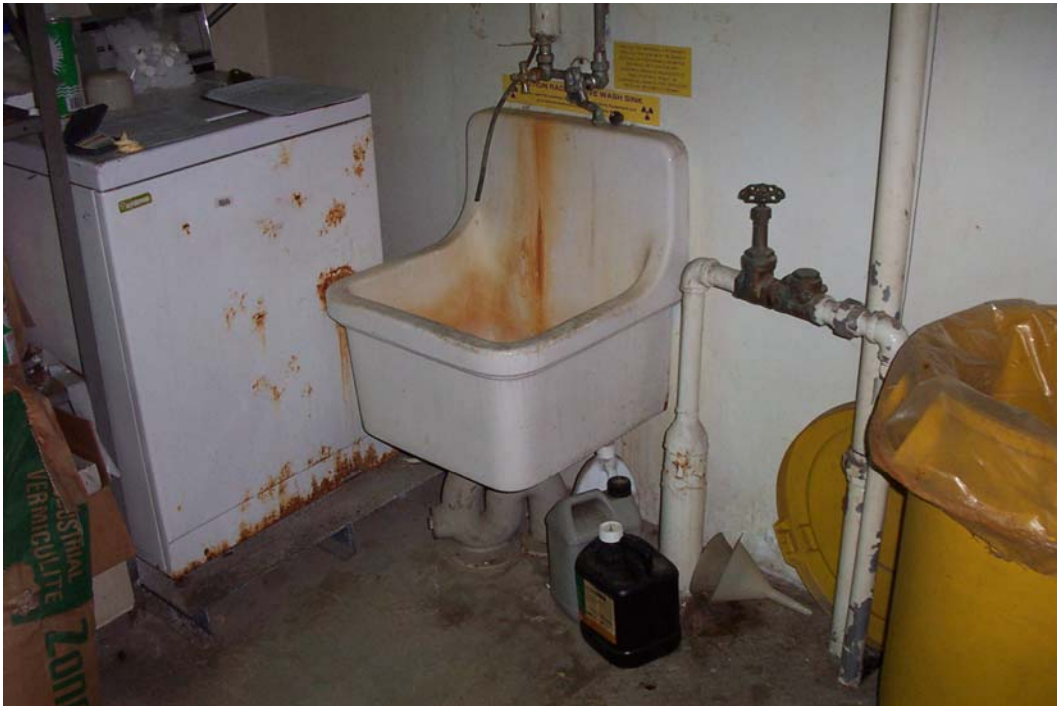
“Warm” Room – Rad Waste Sink
