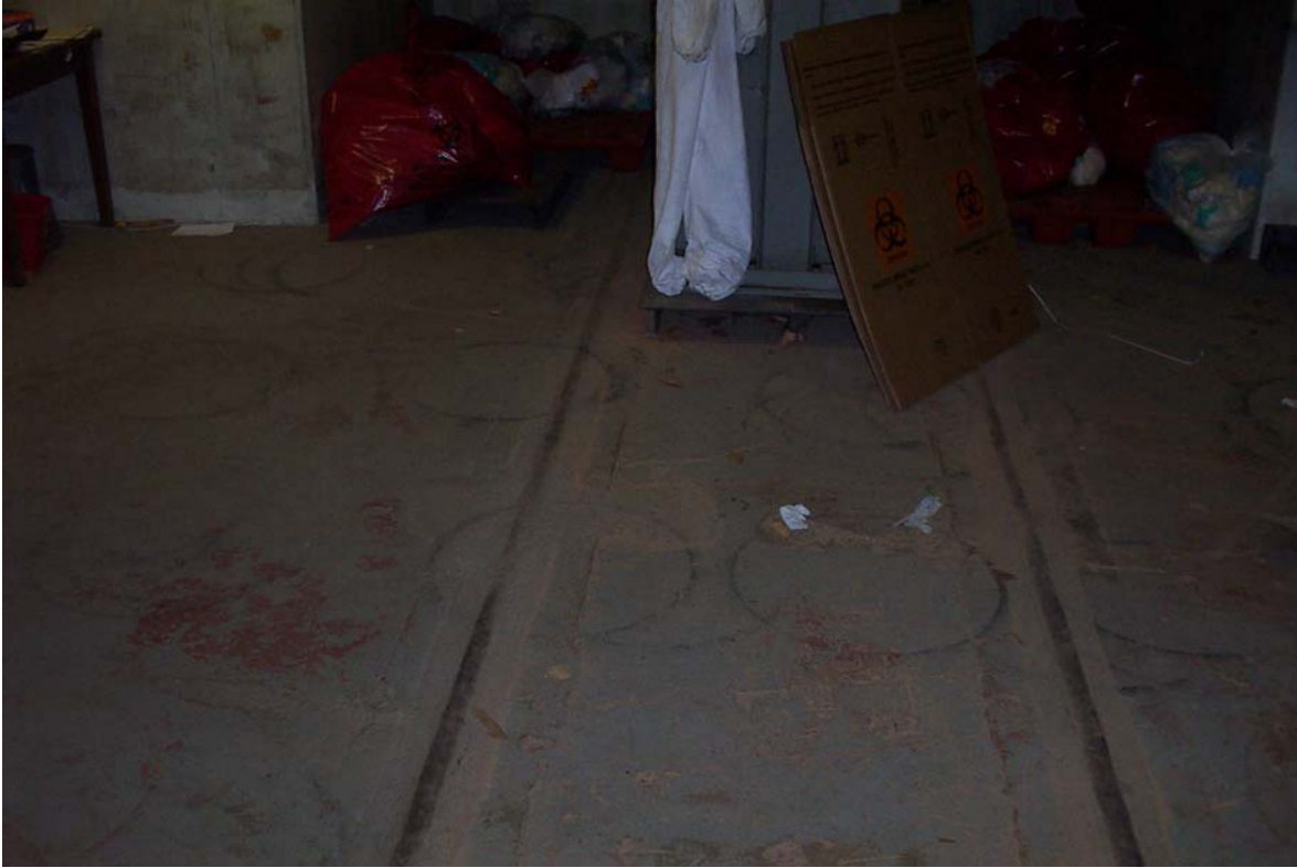
Exposure Room – Track for Former Door
