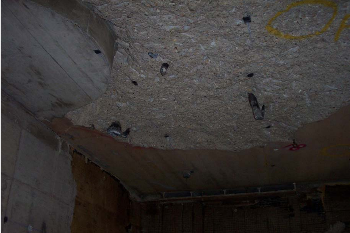
Exposure Room – Ceiling
