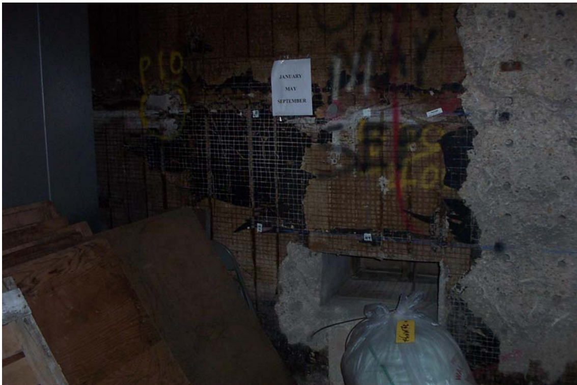
Exposure Room – Nuclear Medicine Clothing Waste (North Wall)
