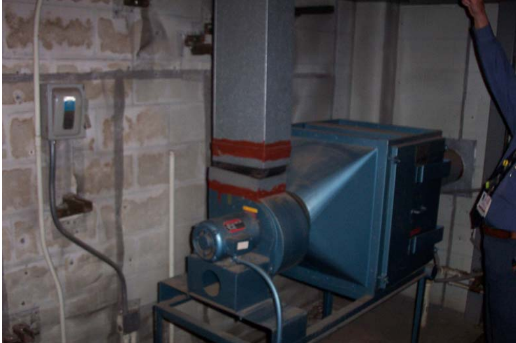
Main Floor – Vial Crusher Ventilation (in “Equipment” Room)
