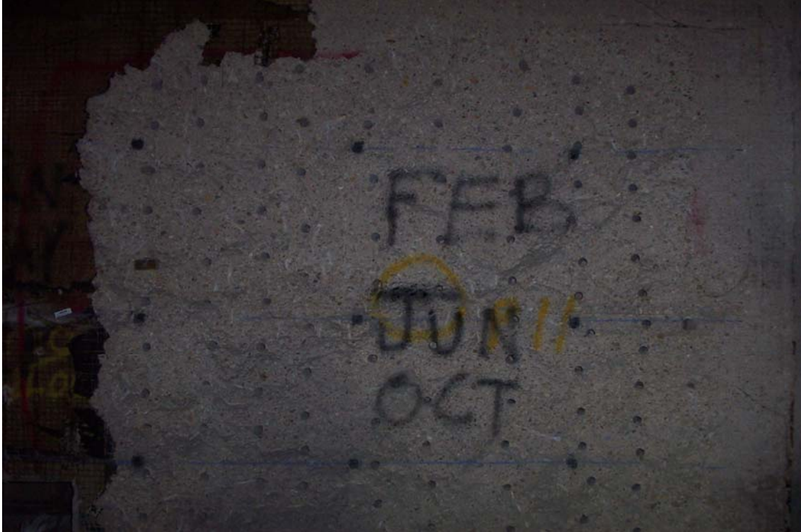
Exposure Room – Concrete Cores and Scabbling (East Wall)
