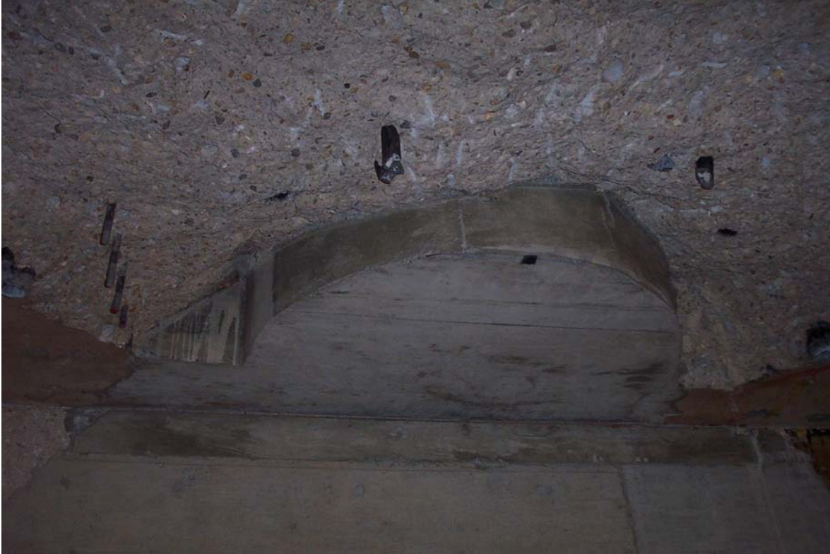
Exposure Room – Ceiling (steel bars)
