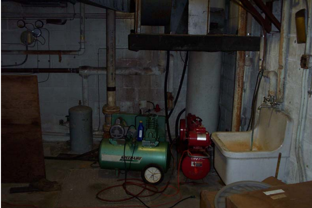
Main Floor – “Equipment” Room
