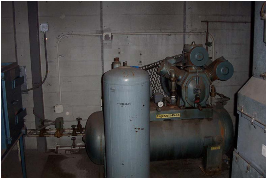
Main Floor – Generator (in “Equipment” Room)
