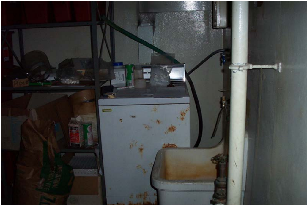
“Warm” Room – Rad Waste Sink
