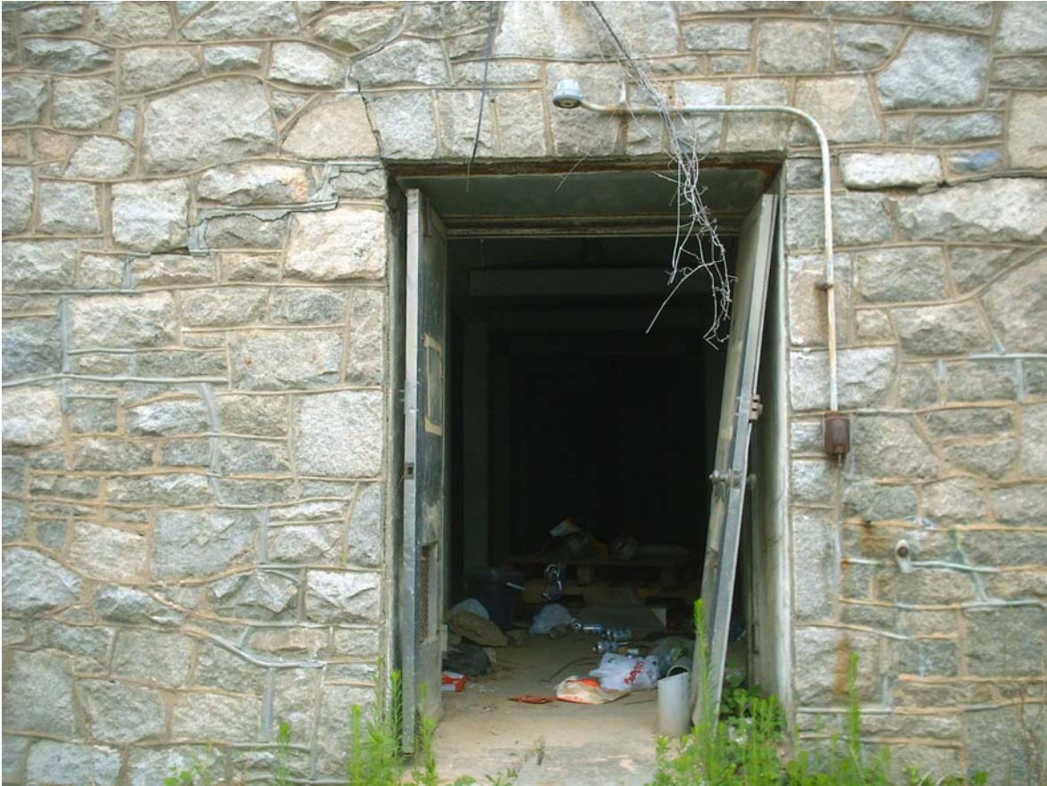
Entrance to Storage Bunker (in side of hill)
