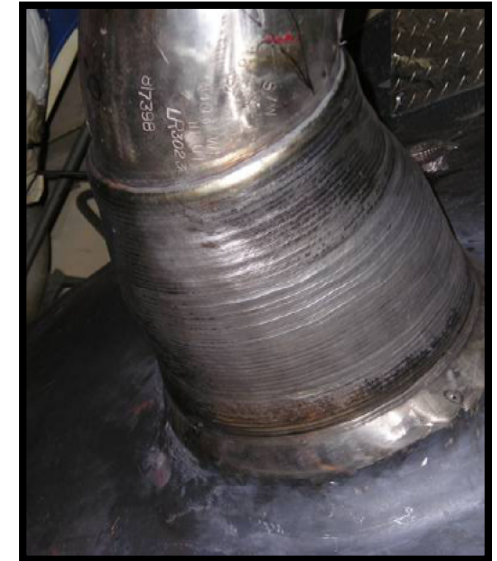
In-process 52M Overlay on Pressurizer Safety Nozzle
