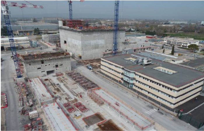
COMURHEX II construction
