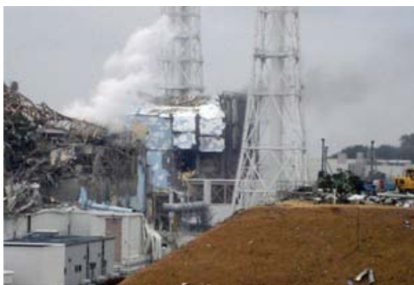
The remnants of reactor No. 1 (left) and No.2's buildings following the explosions.
