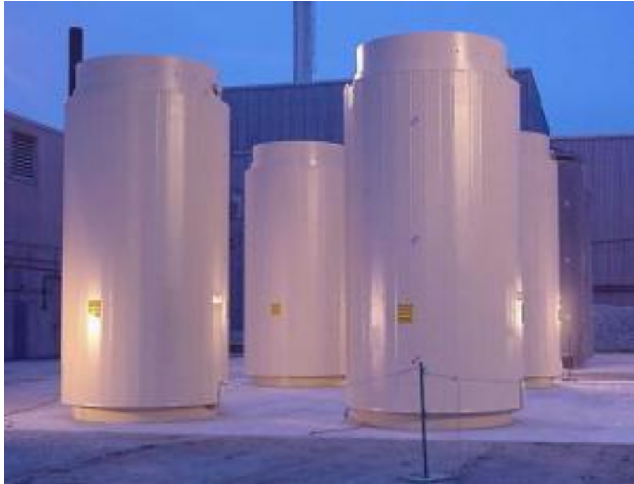
Figure 2. ISFSI at the Dresden Nuclear Power Plant Source: Holtec International Web site
