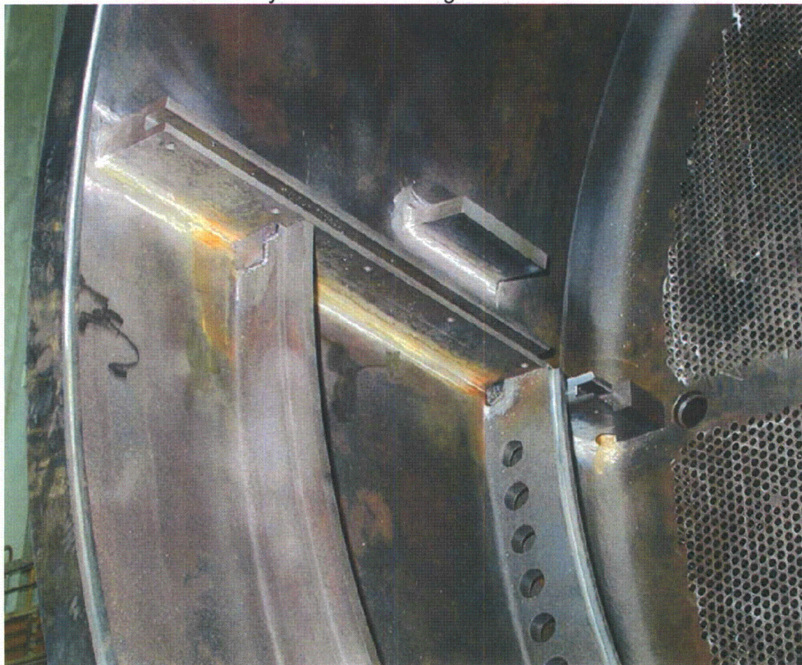
Figure 4 View of Secondary Divider Plate Lugs before Divider Plate Installation
