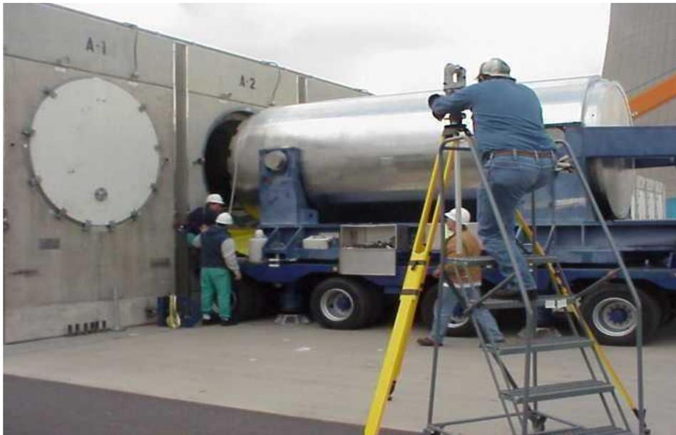
**Figure 1. Horizontal dry cask storage at Susquehanna.**
