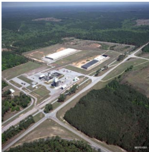
Figure 4.35 Saltstone Manufacturing Facility
