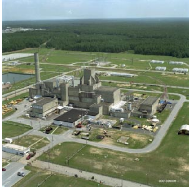
Figure 4.5 C Reactor Facilities
