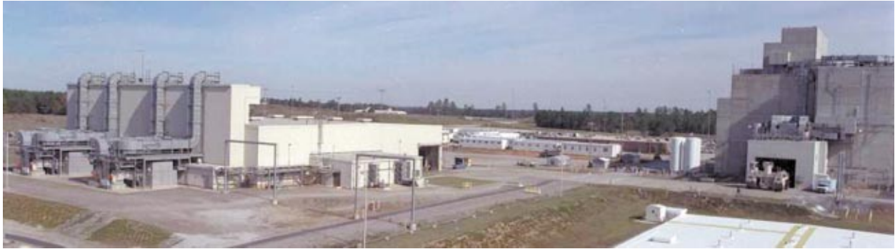
Figure 4.29 High-Level Waste is stabilized in glass in the Defense Waste Processing Facility (right). Canisters containing the glass are stored below ground in the Glass Waste Storage Building (left).
