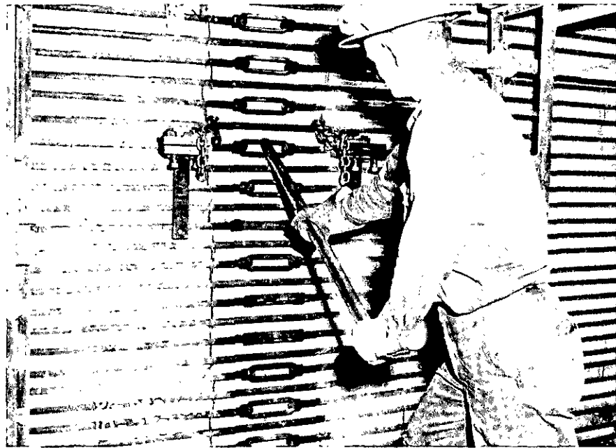
EXHIBIT X-B TENSIONING PROCESS WITH TENSIONING LEVER AT TURNBUCKLES
