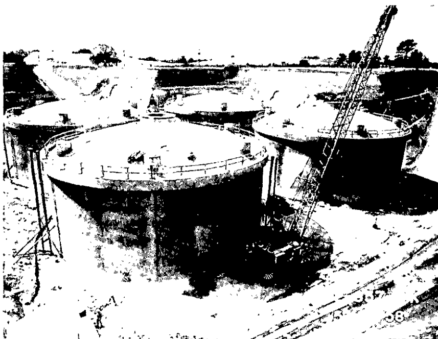
EXHIBIT XII-B COMPLETED TANKS SHOWING PILES NEAR TANK WALL PLACED PRIOR TO BACKFILLING
