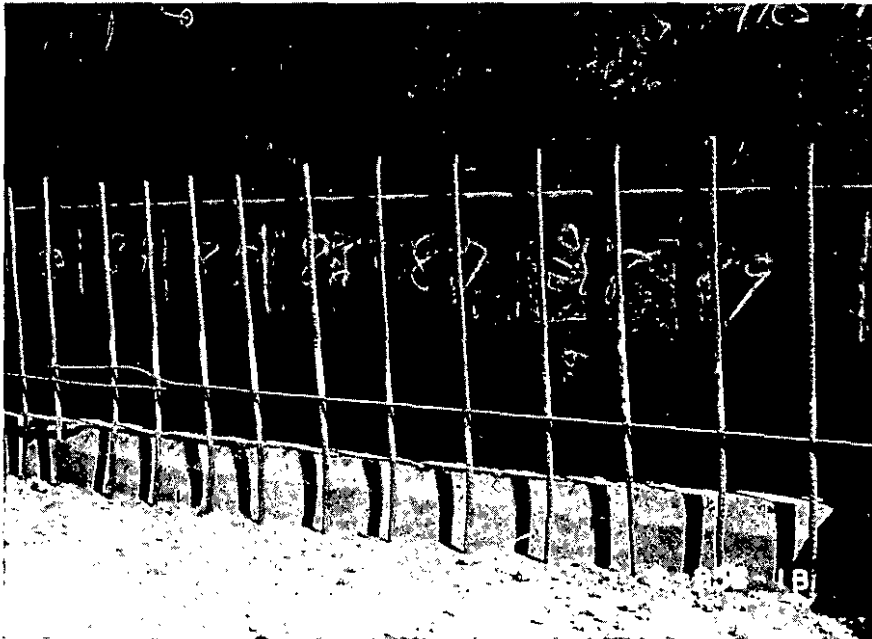
EXHIBIT VII-B OUTSIDE OF STEEL LINER SHOWING KNUCKLE PLATE, WALL FOUNDATION AND DOWELS
