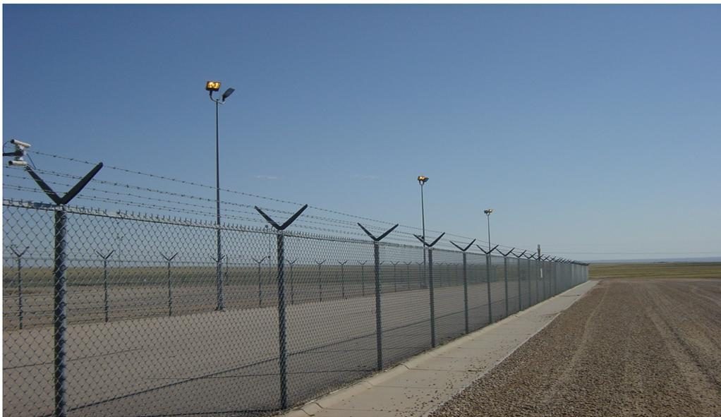
**Figure 73: An example of a perimeter with controlled lighting.**
