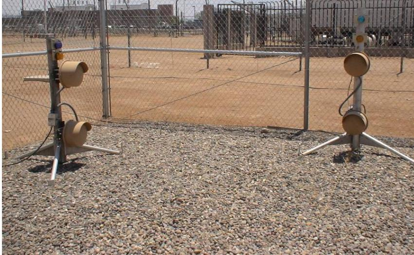
**Figure 5: Example of a corner setup of microwave sensors that provides overlap to decrease the possibility of an adversary crawling beneath the beams.**
