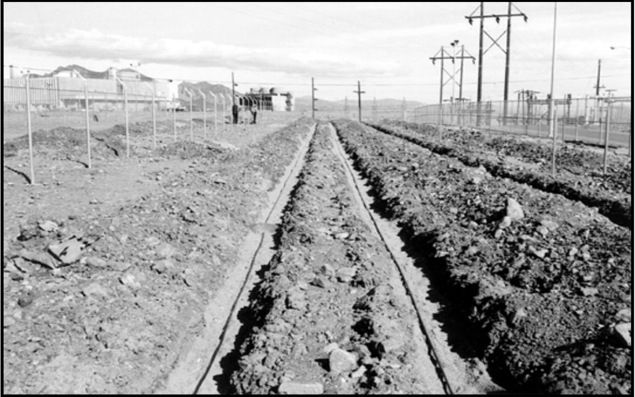
**Figure 20: Typical ported coax cable system installation.**
