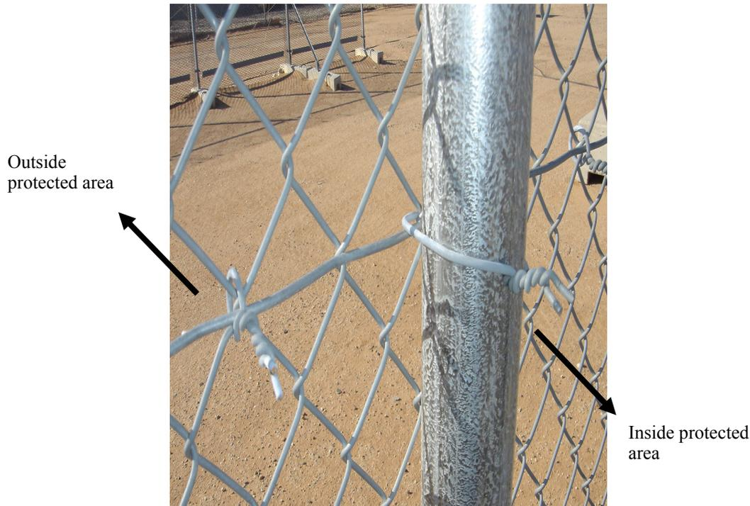
**Figure 33: Example of security fence wire ties.**
