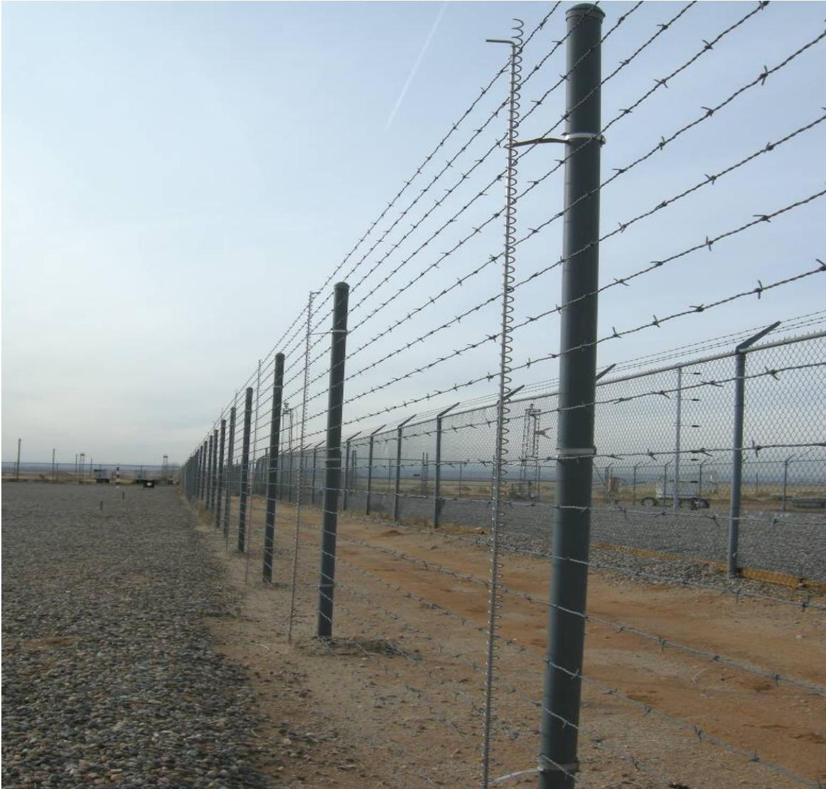
***Figure 26: A freestanding taut wire installation for environmental testing.***
