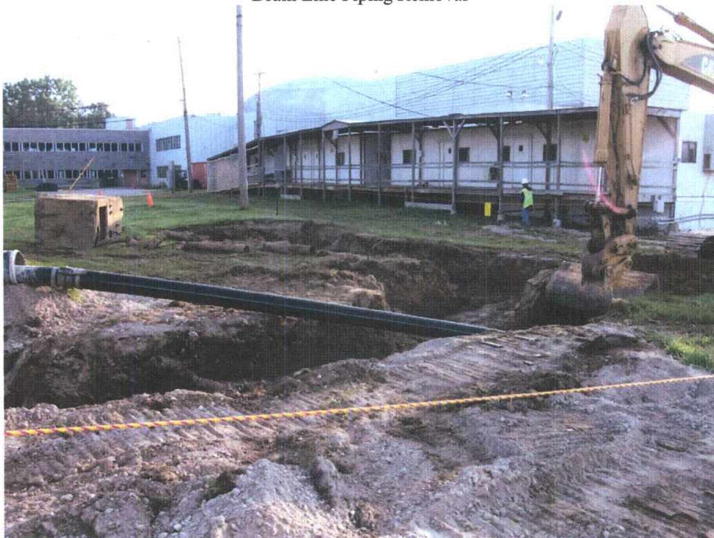
Drain Line Piping Removal
