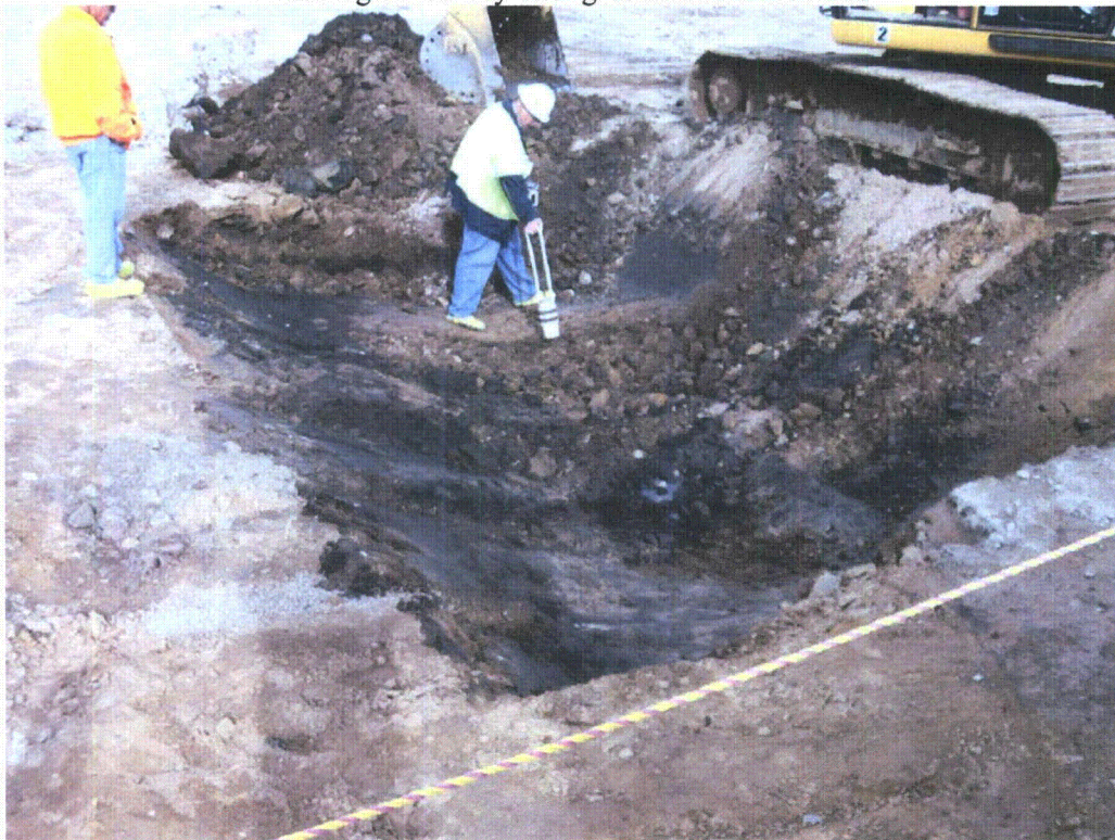
Radiological Survey during Excavation Activities
