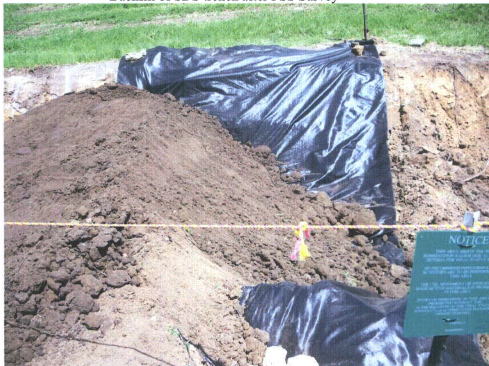
Backfill of SDS trench after FSS Survey
