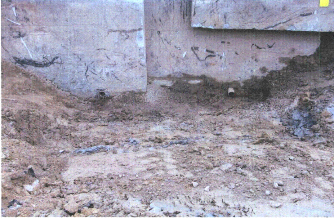
Piping Discovered during FPR walk-down of Trenches North of SEB prior to FSS
