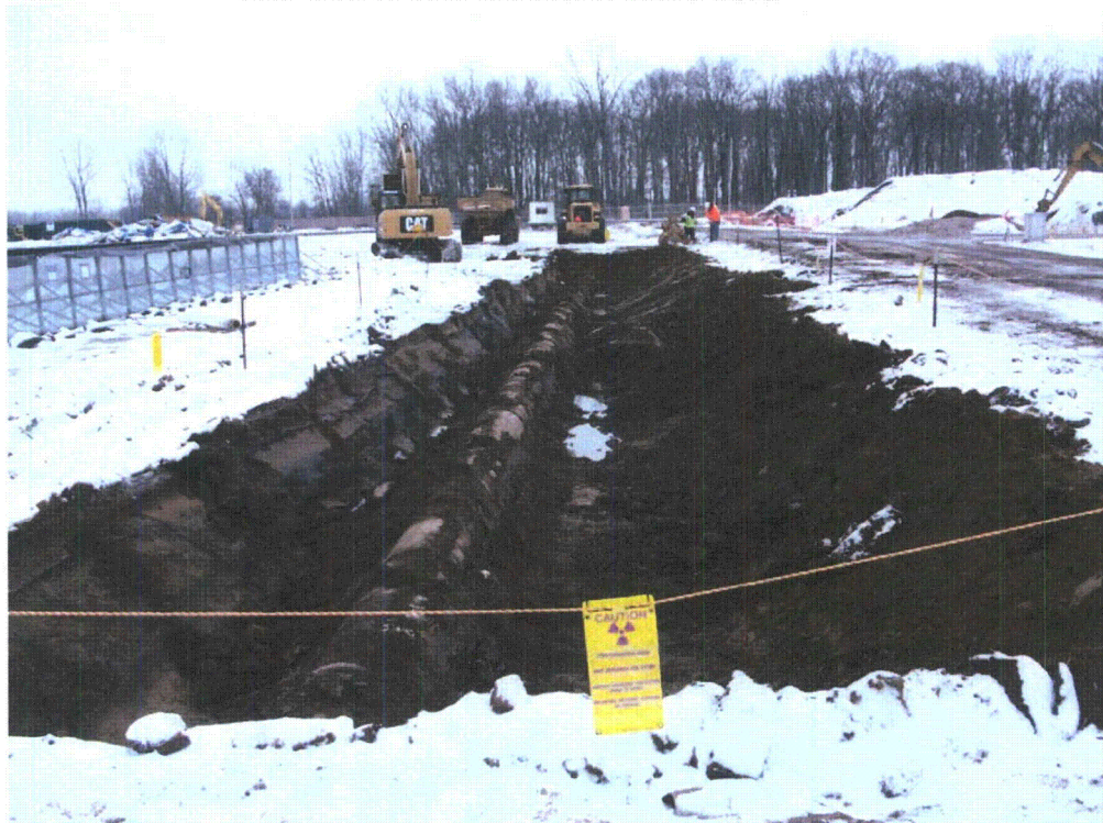
SDS piping removal
