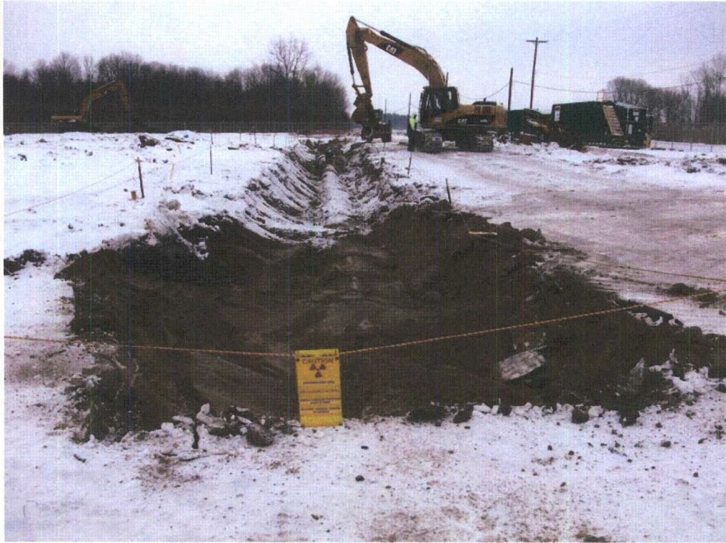
SDS Piping Removal
