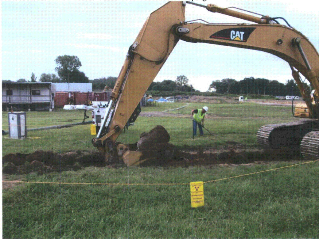
Trench after SDS Piping Removal
