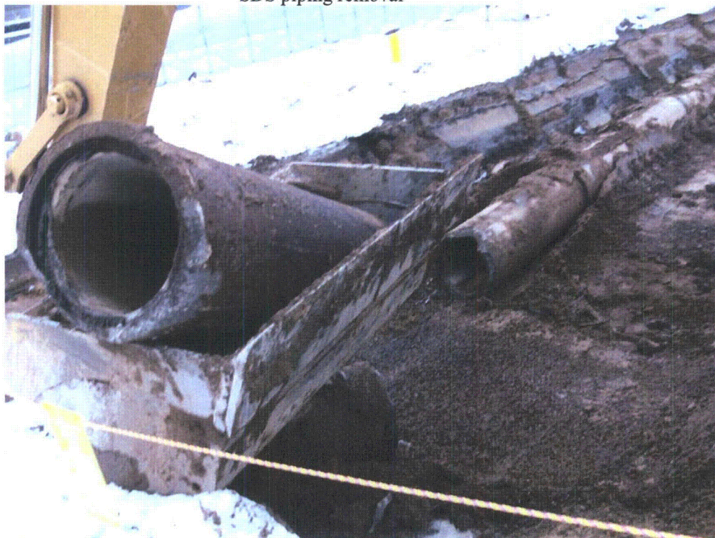
SDS piping removal
