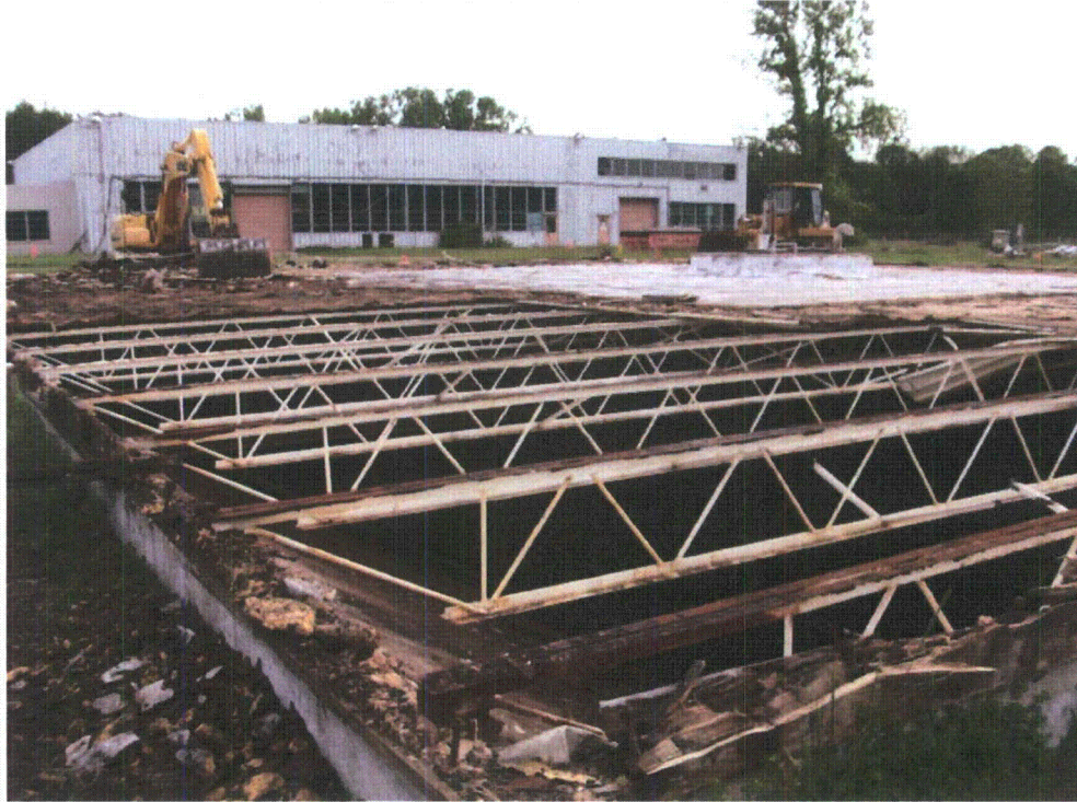
South CRB Concrete Demolition
