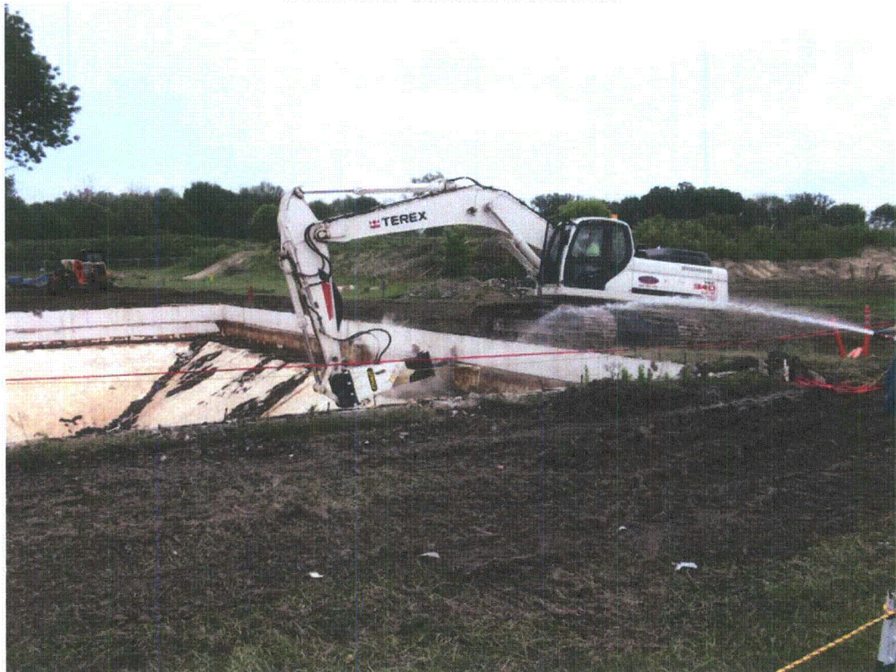
South CRB Concrete Demolition
