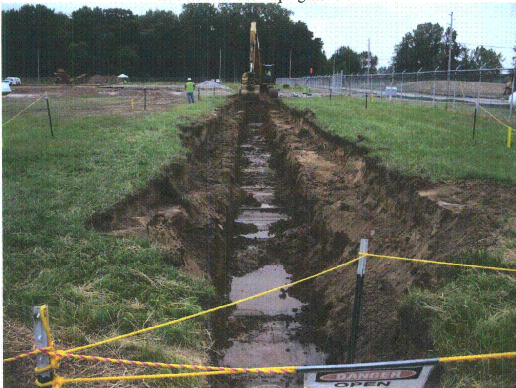
Trench after SDS Piping Removal
