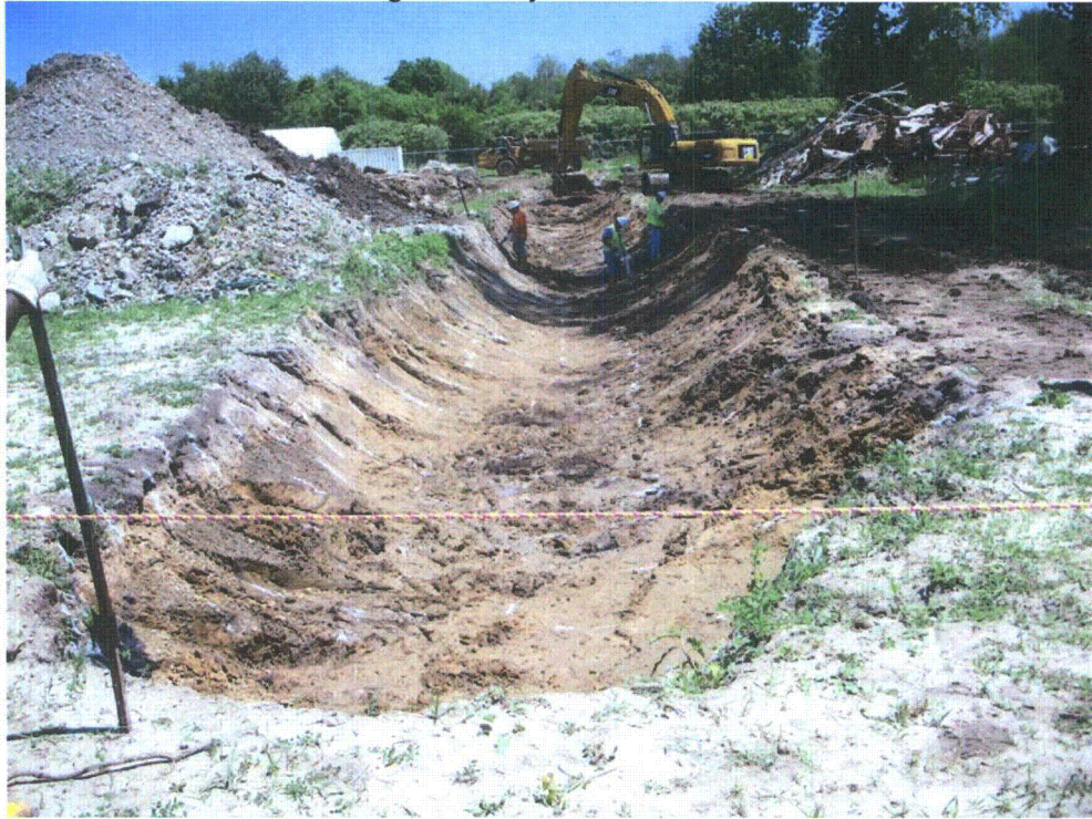
Backfill of SDS trench after FSS Survey
