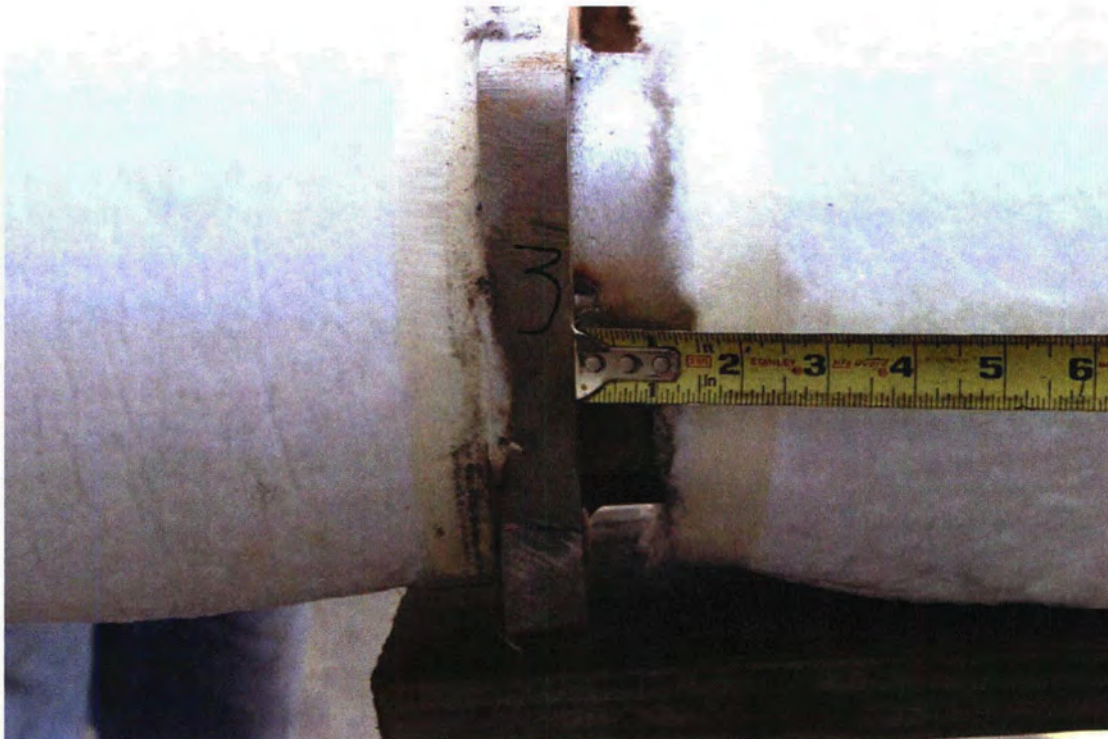
Figure 2.12.2-24 - Insulation Gap at Rib #3
