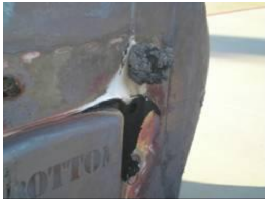
Figure 2.12.1-55 – Foam char in lock pin area
