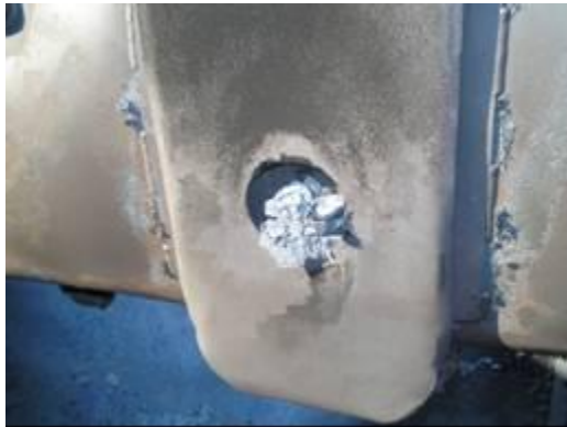
Figure 2.12.1-53 – Vent at stiffener
