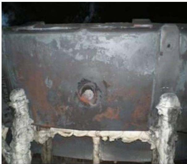
View of Puncture Bar Damage Area
