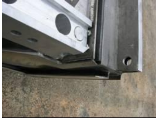
Figure 2.12.1-25 – Cracked top weld
