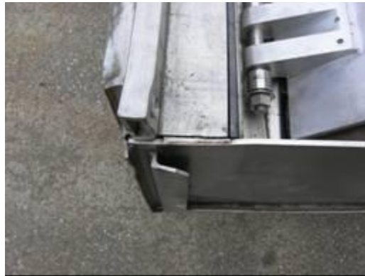
Figure 2.12.1-27 – Cracked bottom weld
