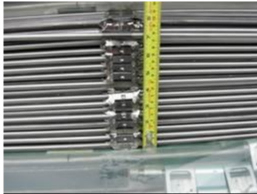
Figure 2.12.1-33 – Mid-span lattice compression
