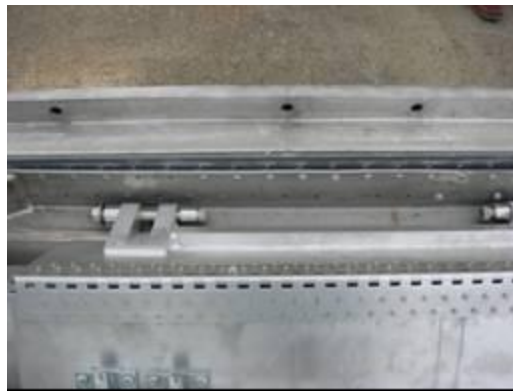
Figure 2.12.1-23 – Location of broken rivets
