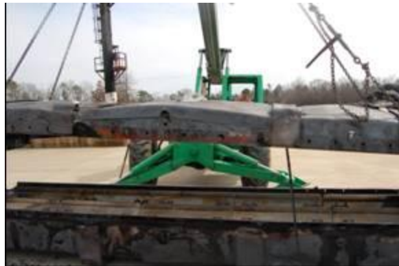
Figure 2.12.1-56 – CTU3 lid removal
