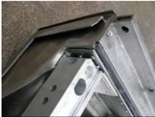
Figure 2.12.1-26 – Cracked top weld
