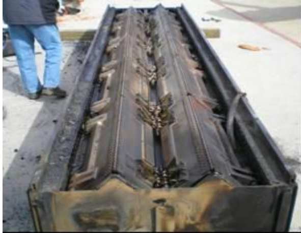
View of Fuel Cavity Doors
