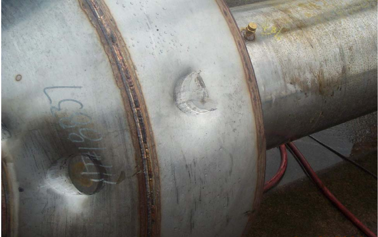
Figure 2.12.4-6 – ETU Test 2: View of Puncture Damage; ~3/4" Deep
