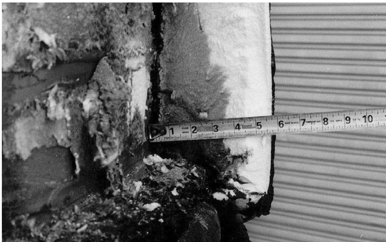
Figure 2.10.3-83 – CTU; Residual Foam in OCA Lid Side; Remote from Test Damage
