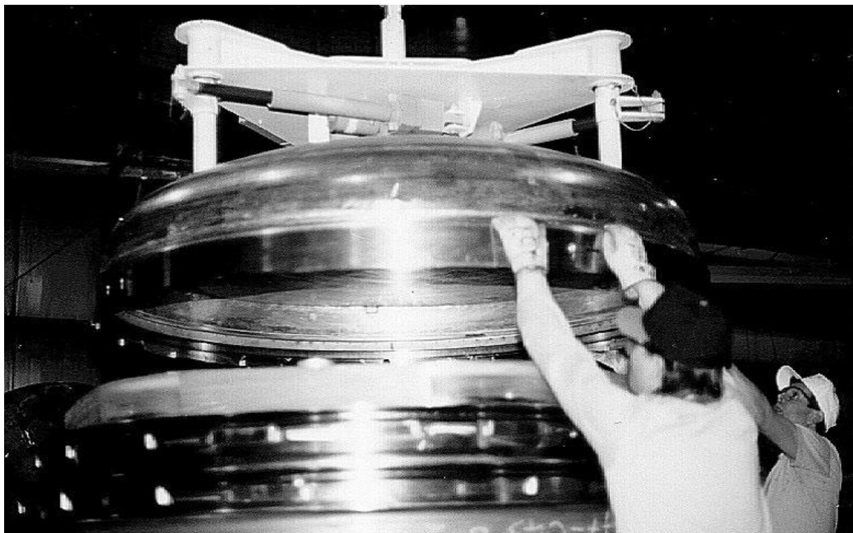
Figure 2.10.3-53 – CTU; Final ICV Lid Alignment During ICV Lid Installation
