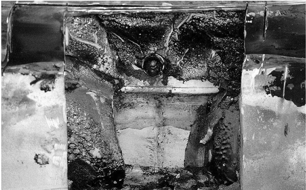
Figure 2.10.3-85 – CTU; OCV Vent Port Region After Removing Excess Foam Char
