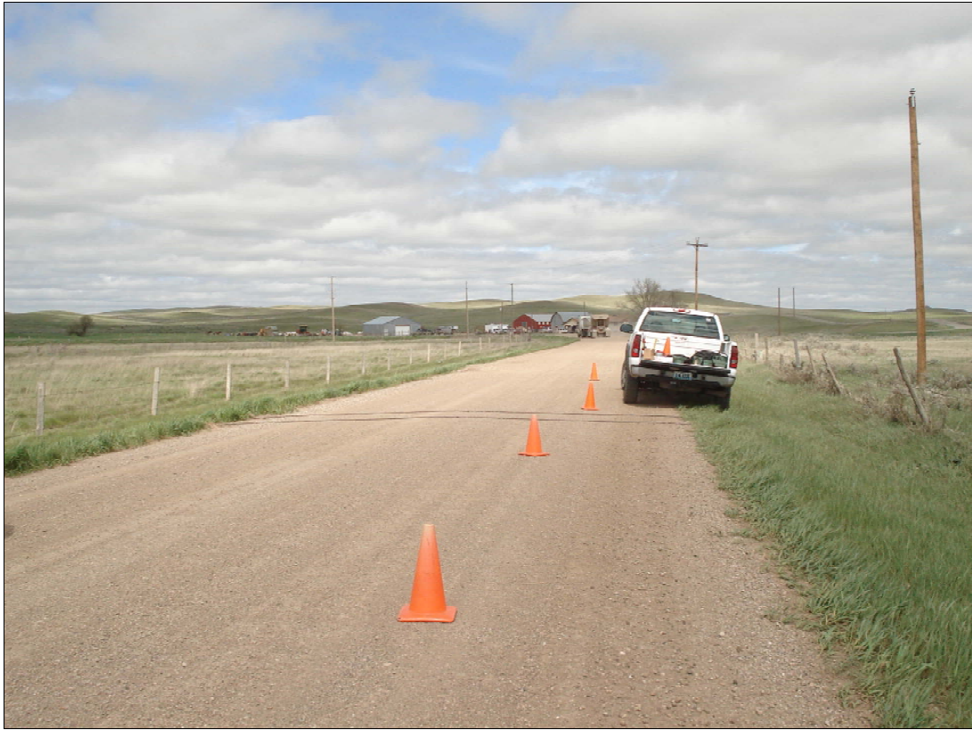
Site 003 Cabin Creek Road Looking West
