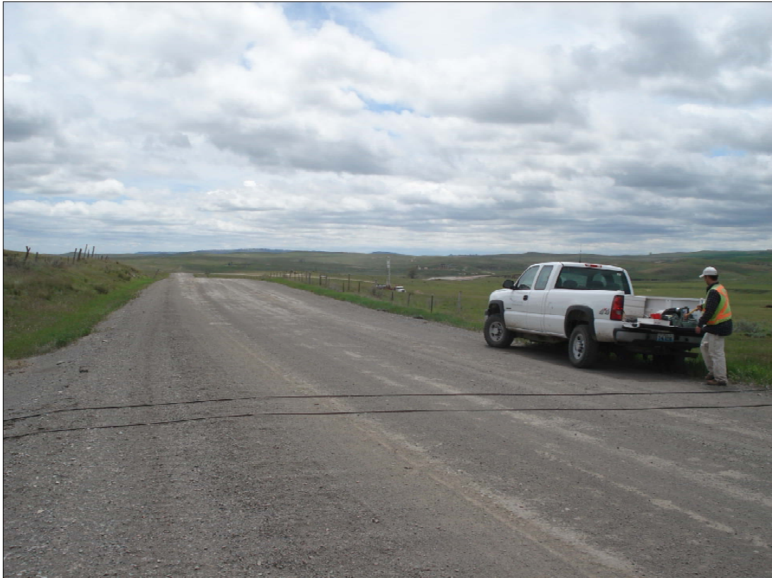
Site 006 D Road Looking Southeast
