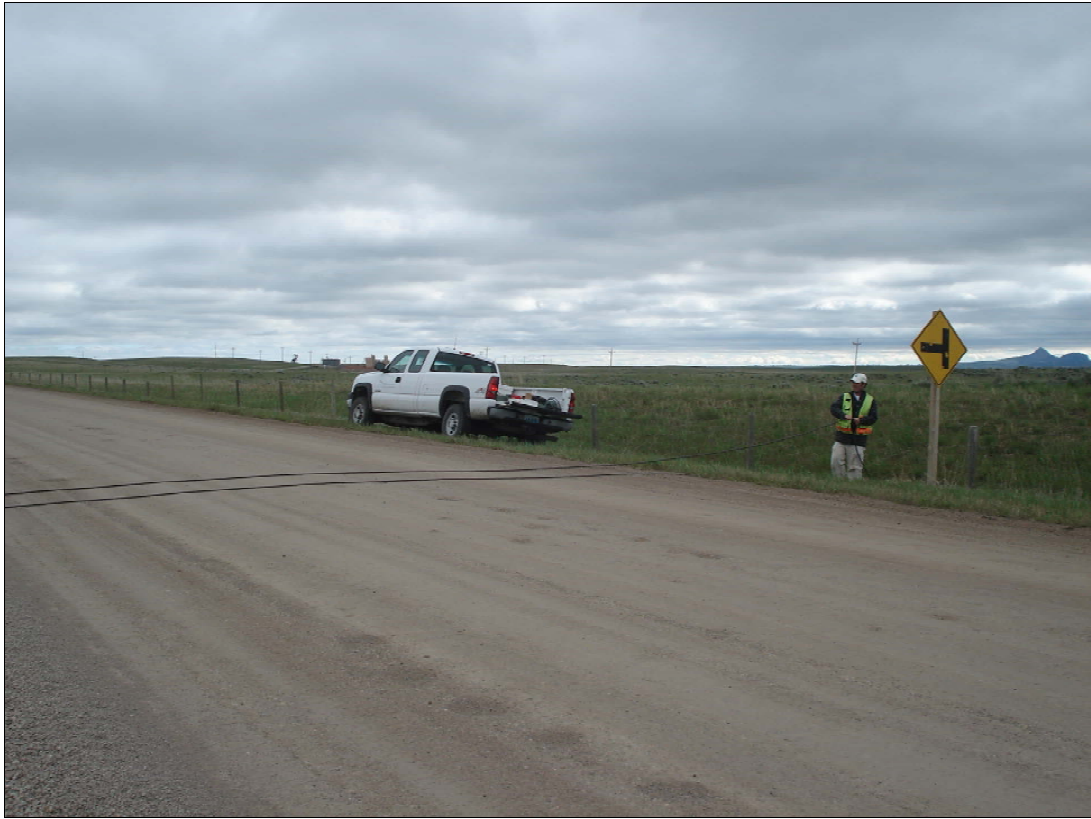
Site 001 New Haven Road Looking North
