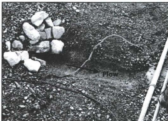
Figure 2.5 Photograph of Unit 2 Moat Drainage to Ground Surface
