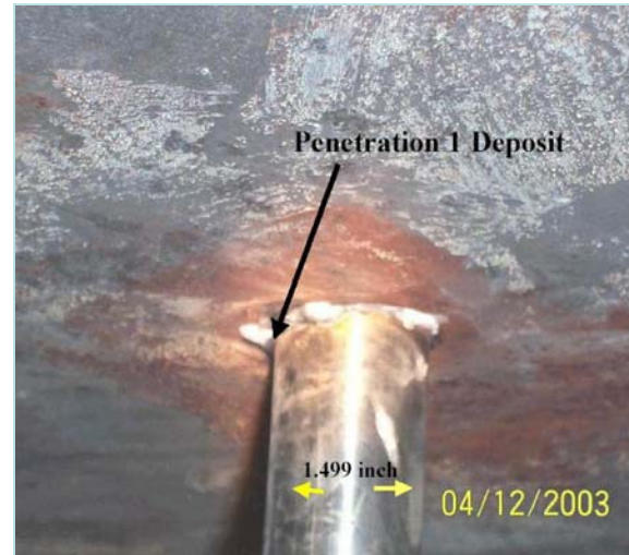
Boric acid white residue on leaking reactor vessel penetration
