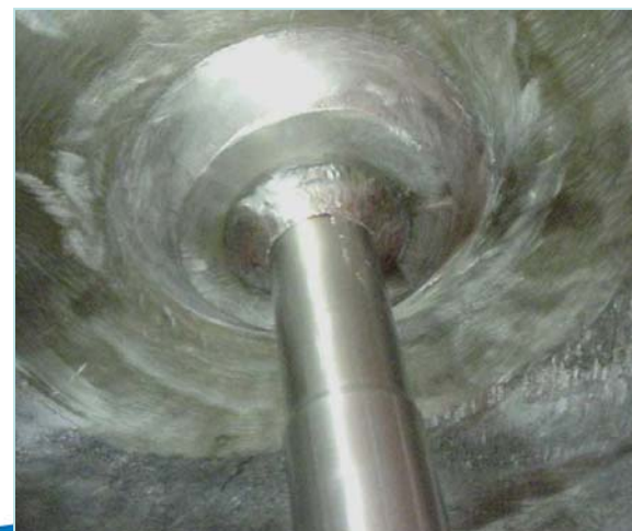
Repaired reactor vessel penetration
