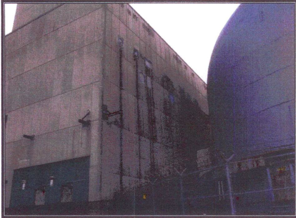
Plate 59 Location of KAPOW! pipes on north wall of steam generator building (Photograph by RCG&A, 2008)
