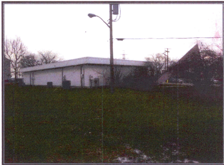
Plate 149 View of visitor's center looking east (Photograph by RCG&A, 2008)
