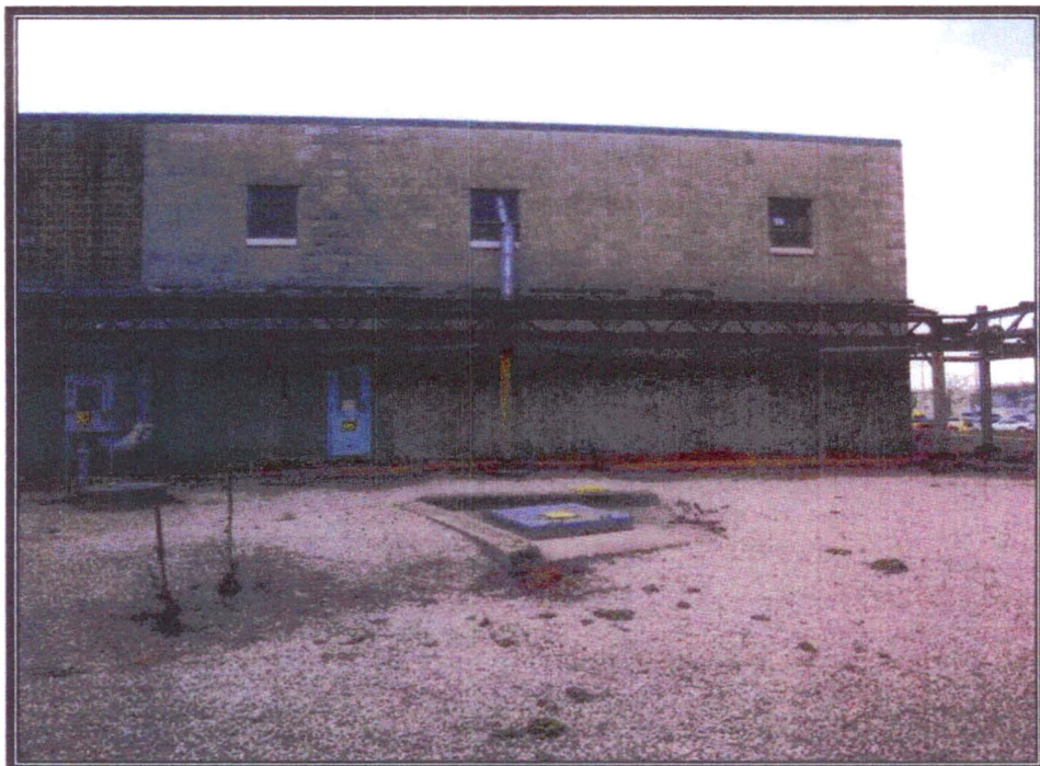
Plate 136 East wall of sodium service building showing upper, concrete block section (Photograph by RCG&A, 2008)
