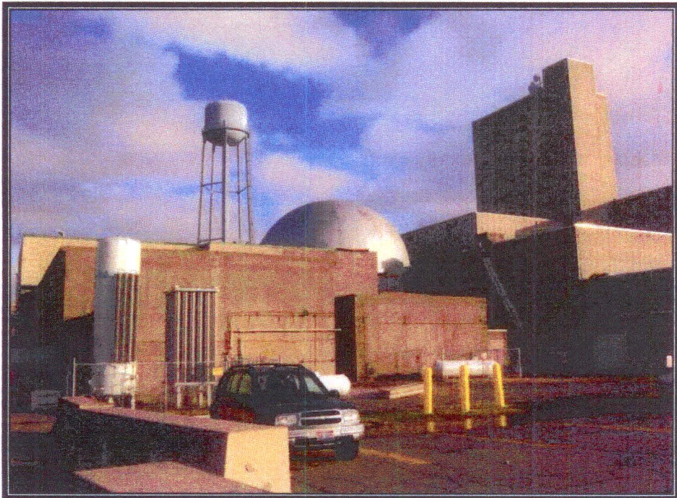
Plate 147 View of plant looking southeast, note water tower (Photograph by RCG&A, 2008)
