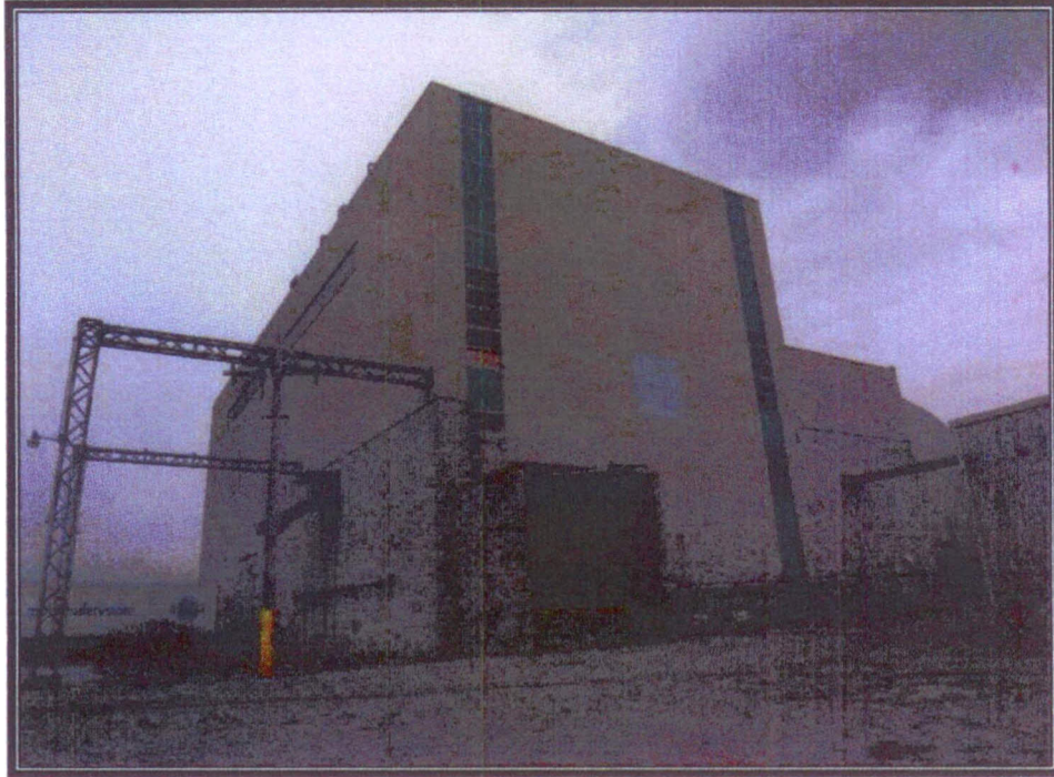
Plate 18 View of turbine building looking northwest (Photograph by RCG&A, 2008)
