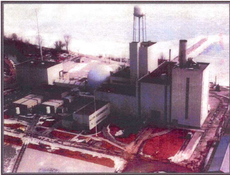
Plate 41 Aerial view of plant showing boiler house to the right, ca. 1975 (Courtesy DECo)
