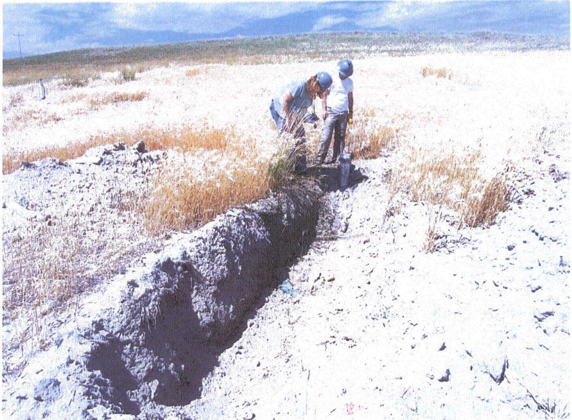
Figure 7 View of un-reclaimed mud
