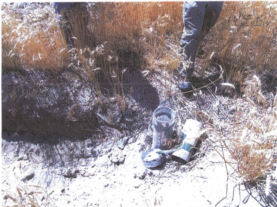
Figure 6 View of possible open hole, broken pipe
