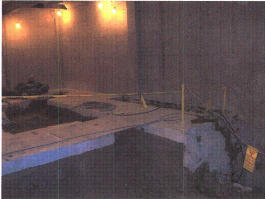
Basement Area Adjacent to Evaporator Pit Where Concrete and Soil Were Removed
