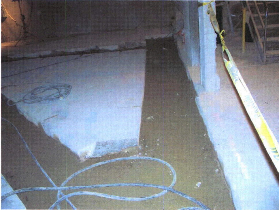
Central Work Area Looking South, Showing Floor Drain Excavations
