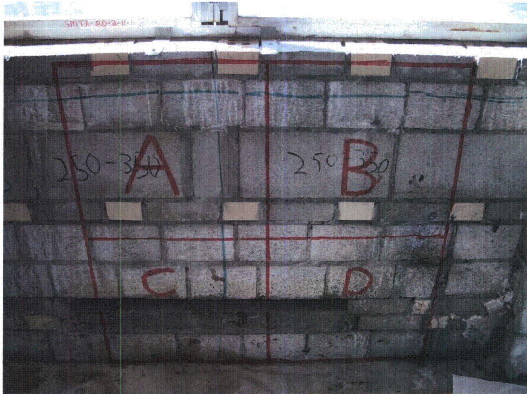
Exhibit 14, Room 213A West Wall Showing Example of a Surface Measurement Test Area (SMTA)
