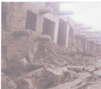
Pilings that were supposed to assure that the building was stable.
