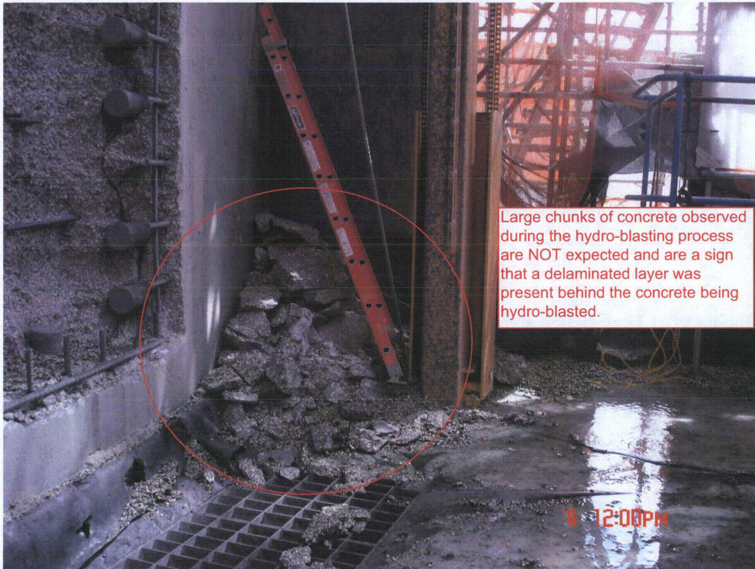
10/4: Cracks at bottom on right side and large chunks of concrete after hydro-blasting
