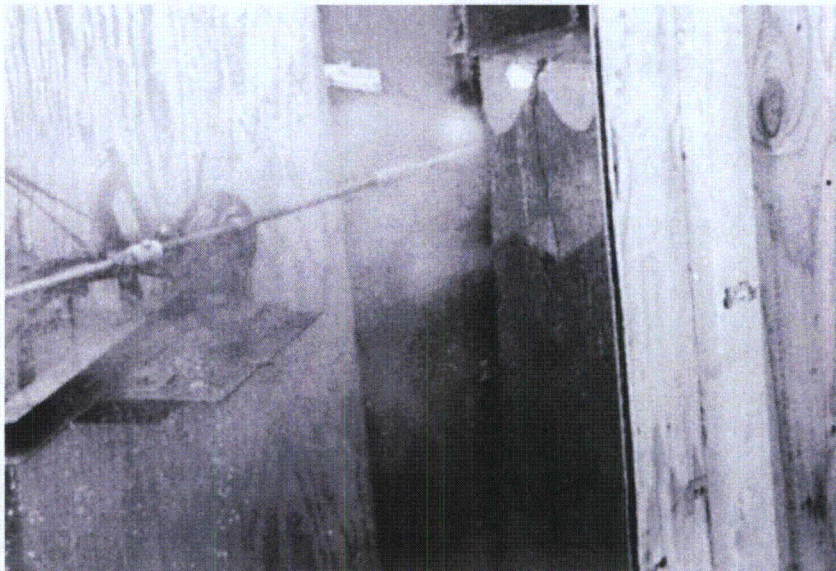
Figure 5.45 Slot cut to make a door at the UMR Rock Mechanics Facility.
