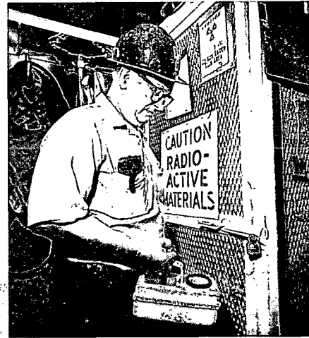
Figure 14. Radiography cameras cannot be left unattended. When not in use, they must be stored in a locked area to prevent unauthorized people from taking the camera. Note the radiographer surveying as he goes to take a camera out of storage. Note also the warning signs that are posted.
