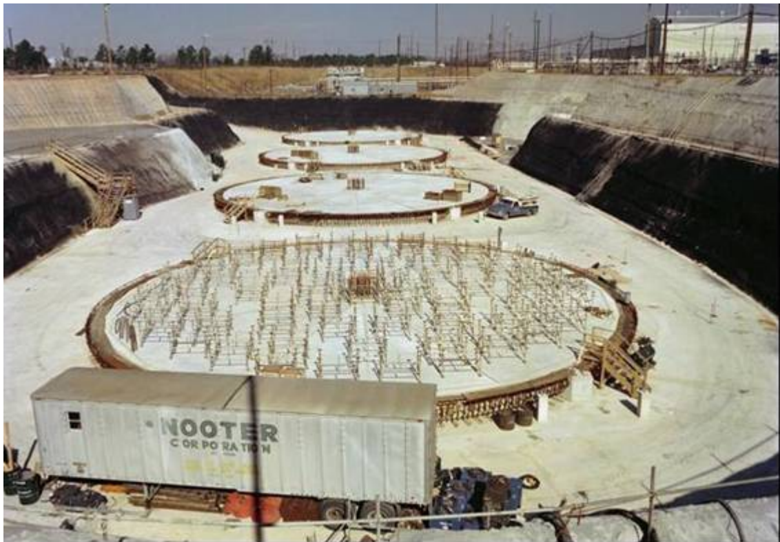
Figure 3.2-20: Scaffolding Set-up on Basemat
