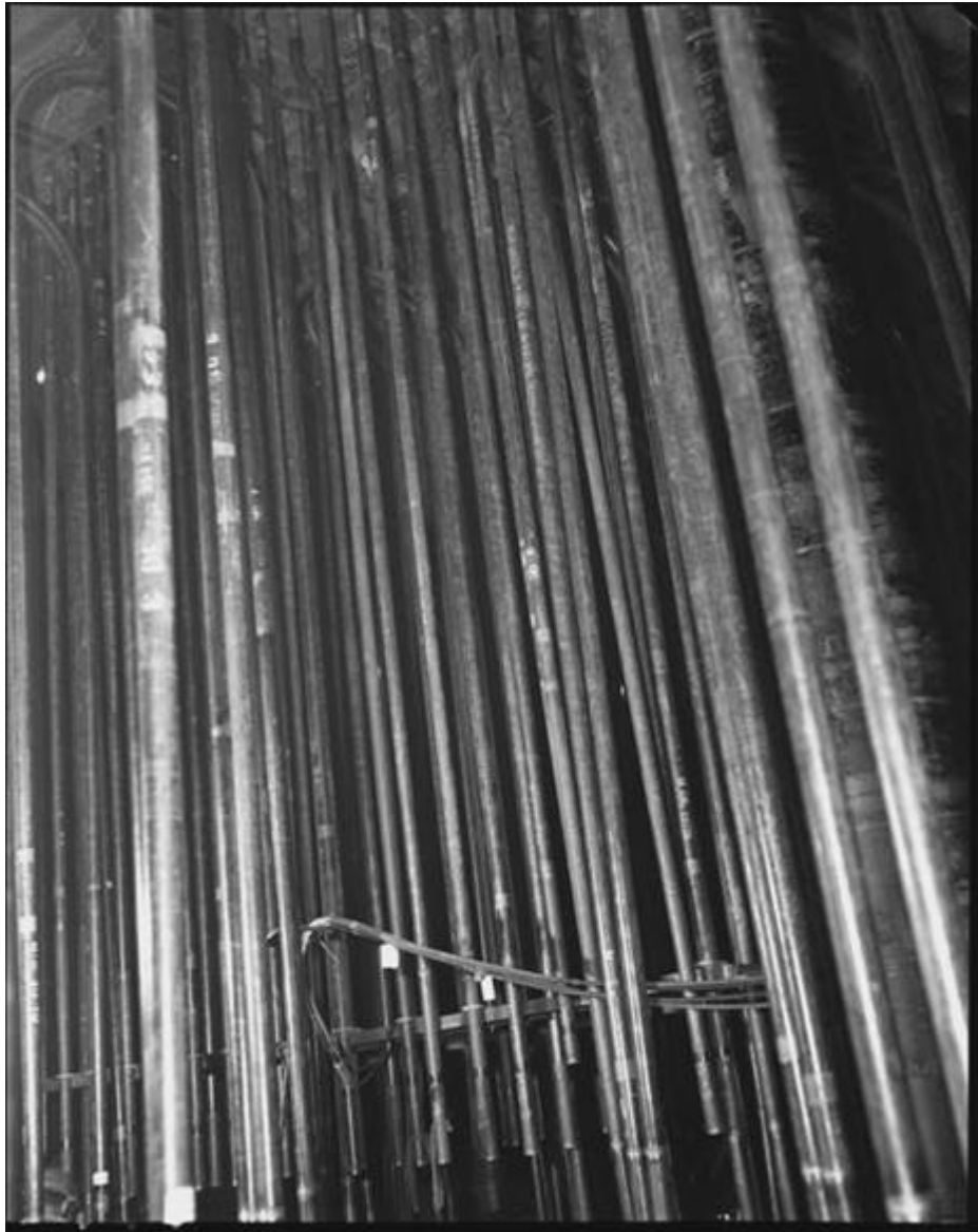
Figure 3.2-12: Type I Tank Cooling Coils During Construction
