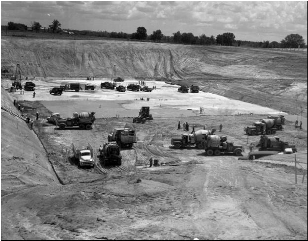
Figure 3.2-3: Tanks 1 through 8 Working Slab Soil Preparation
