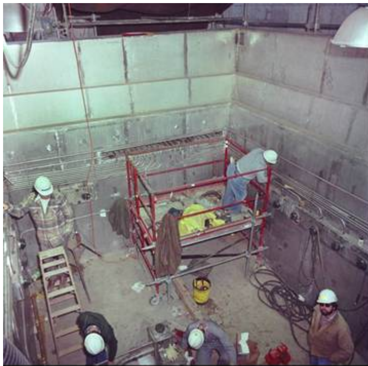
Figure 3.2-58: Diversion Box Stainless Steel Liner Installation
