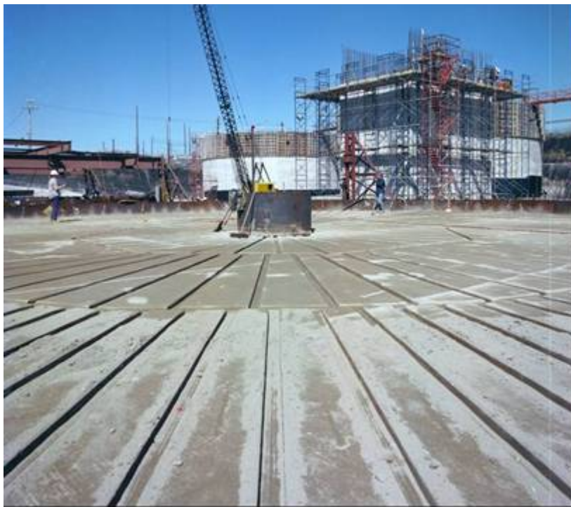
Figure 3.2-22: Radial Air Groove Close-up
