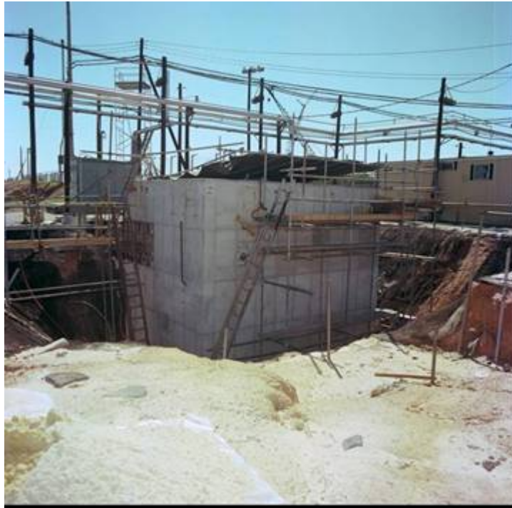
Figure 3.2-57: Diversion Box Later Construction Phase
