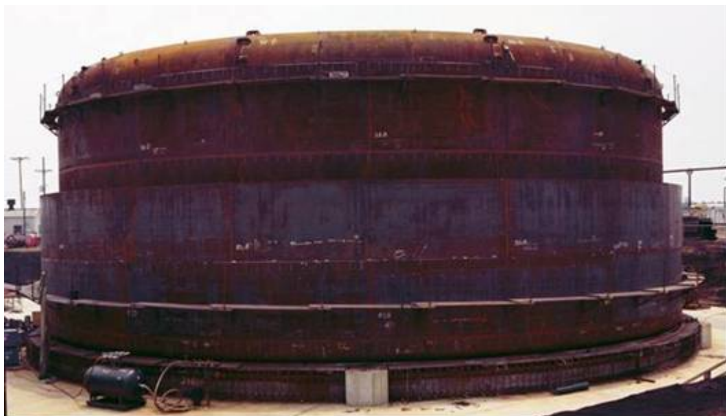
Figure 3.2-19: Type IIIA Tank Primary and Secondary Liner - Late Construction
