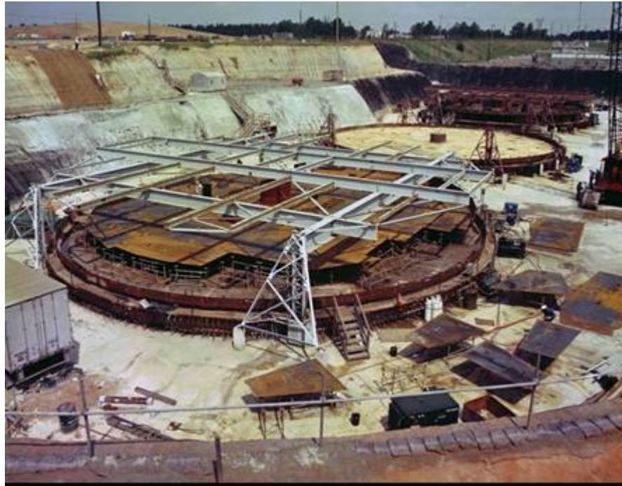
Figure 3.2-18: Type IIIA Tank Primary and Secondary Liner - Early Construction
