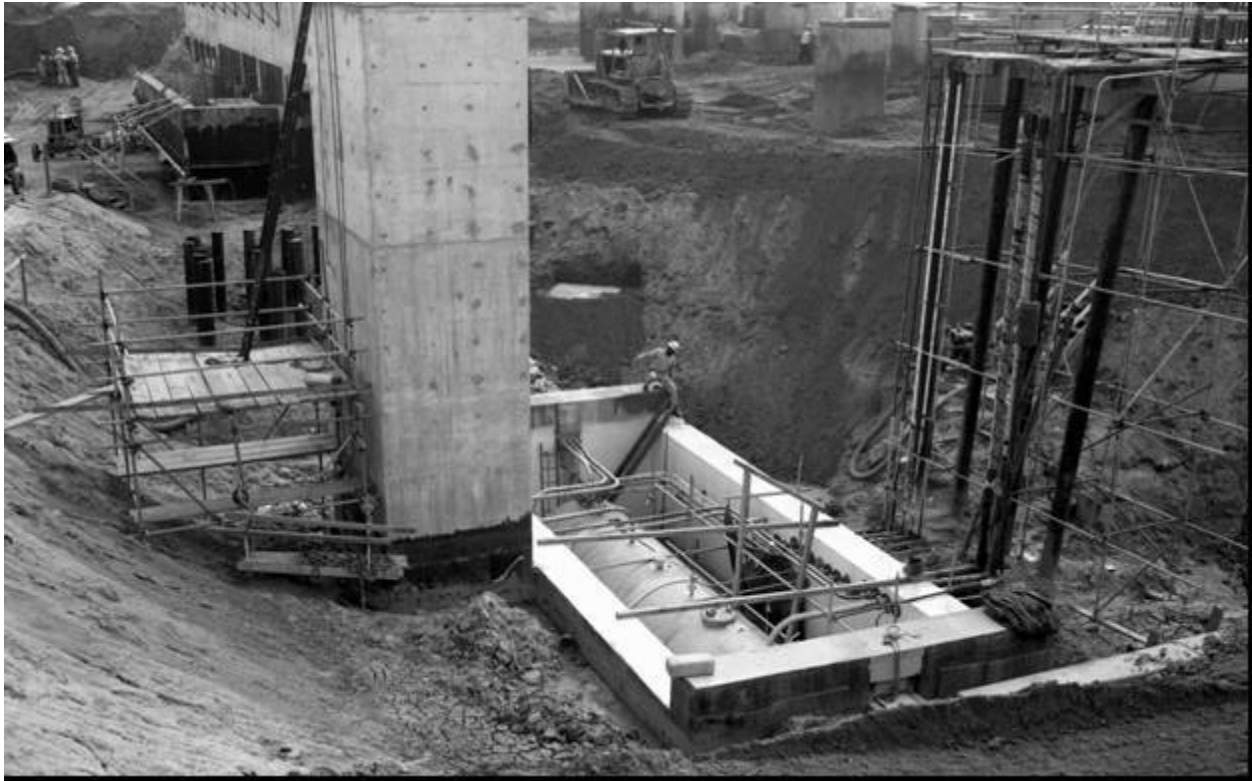
Figure 3.2-48: F-Area Catch Tank During Construction
