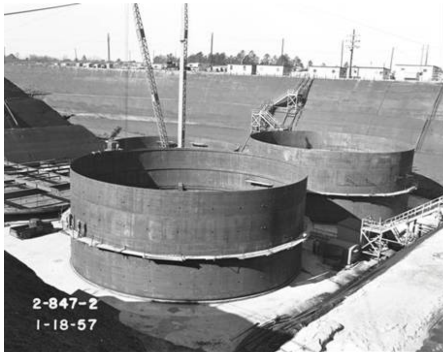
Figure 3.2-33: Construction of the Primary Liners in Type IV Tanks (View 2)
