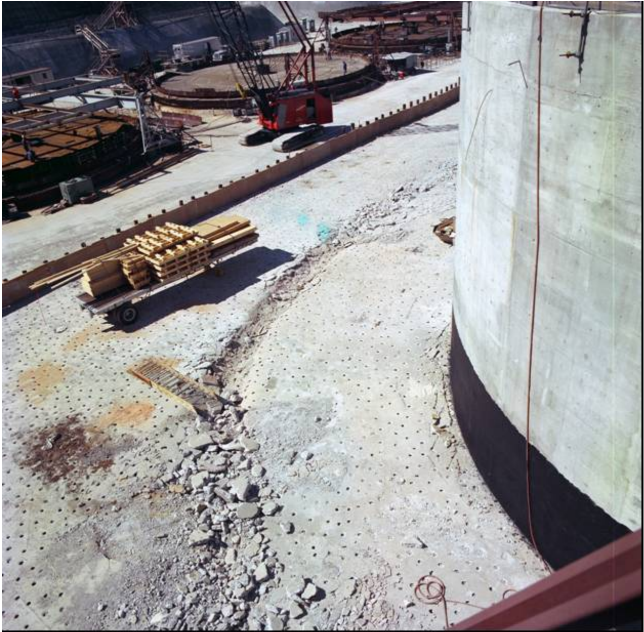
Figure 3.2-26: Drilled Working Slab Around a Type IIIA Tank
