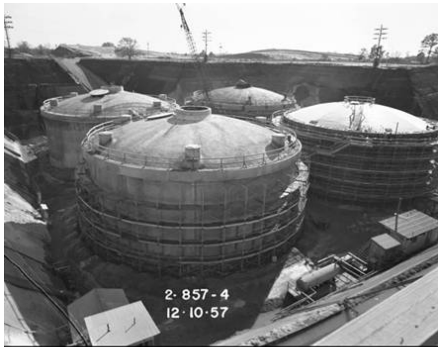
Figure 3.2-34: Dome and Risers on Type IV Tanks
