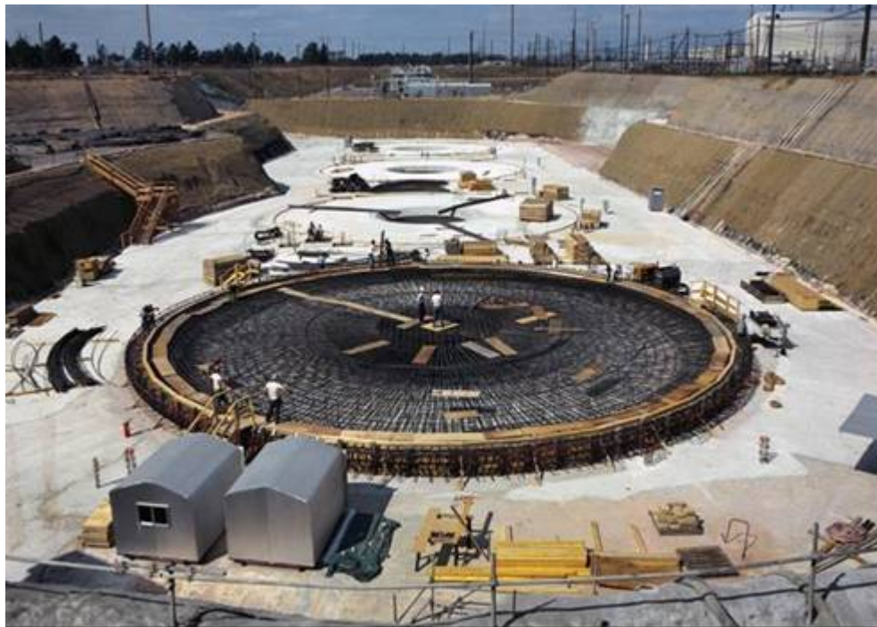
Figure 3.2-16: Early Construction of a Type III/IIIA Tank Basemat
