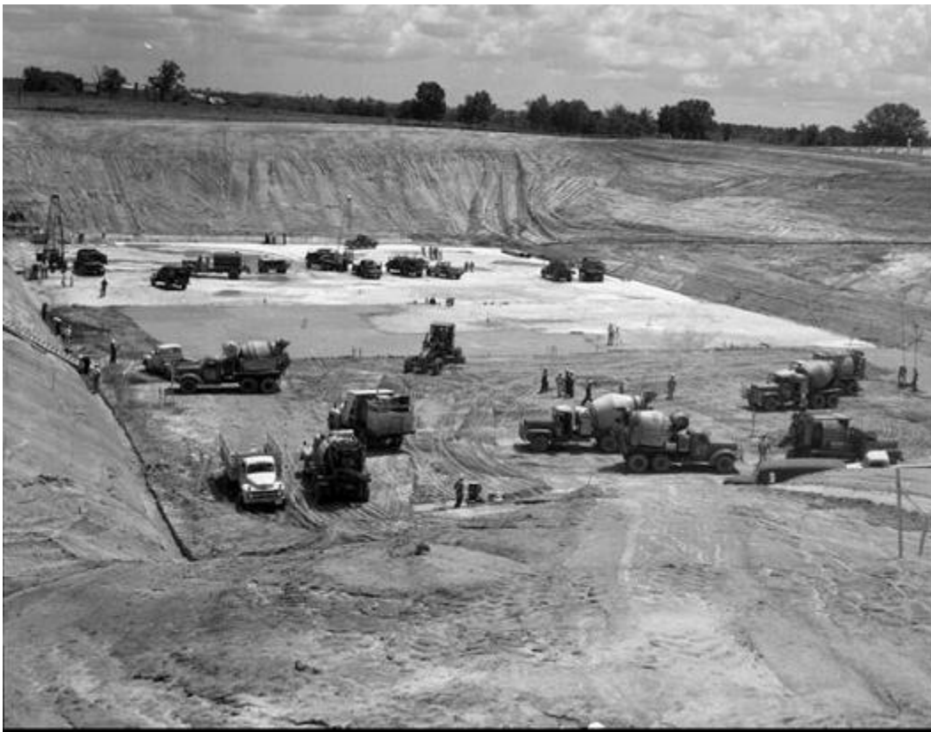
Figure 4.2-21: Tanks 1 – 8 Working Slab
