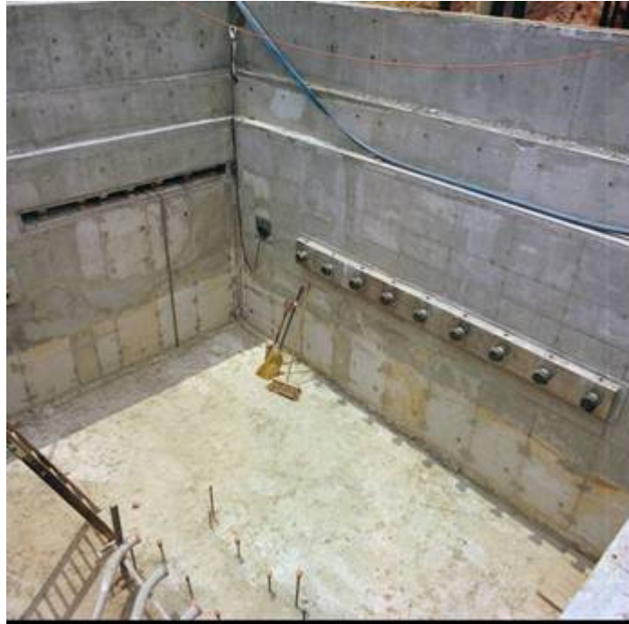
Figure 3.2-54: FDB-4 Concrete Vault During Construction (View 1)
