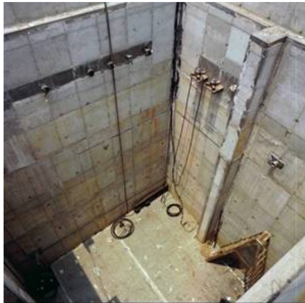
Figure 3.2-43: FPP-2 Concrete Vault During Construction (View 1)
