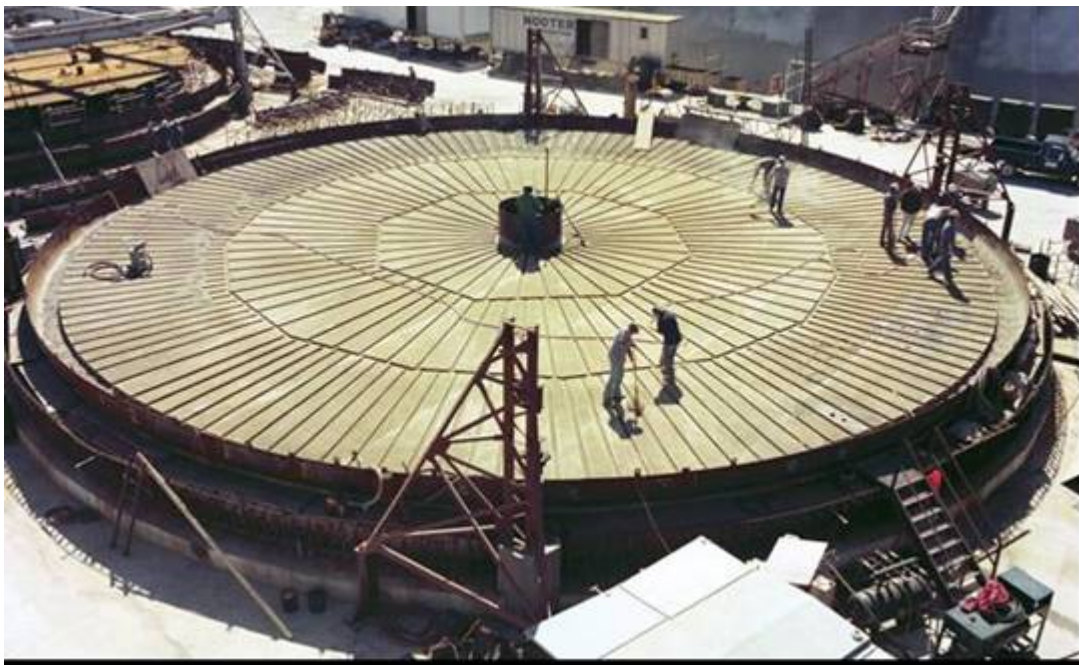
Figure 3.2-21: Radial Air Grooves for Type III/IIIA Tanks
