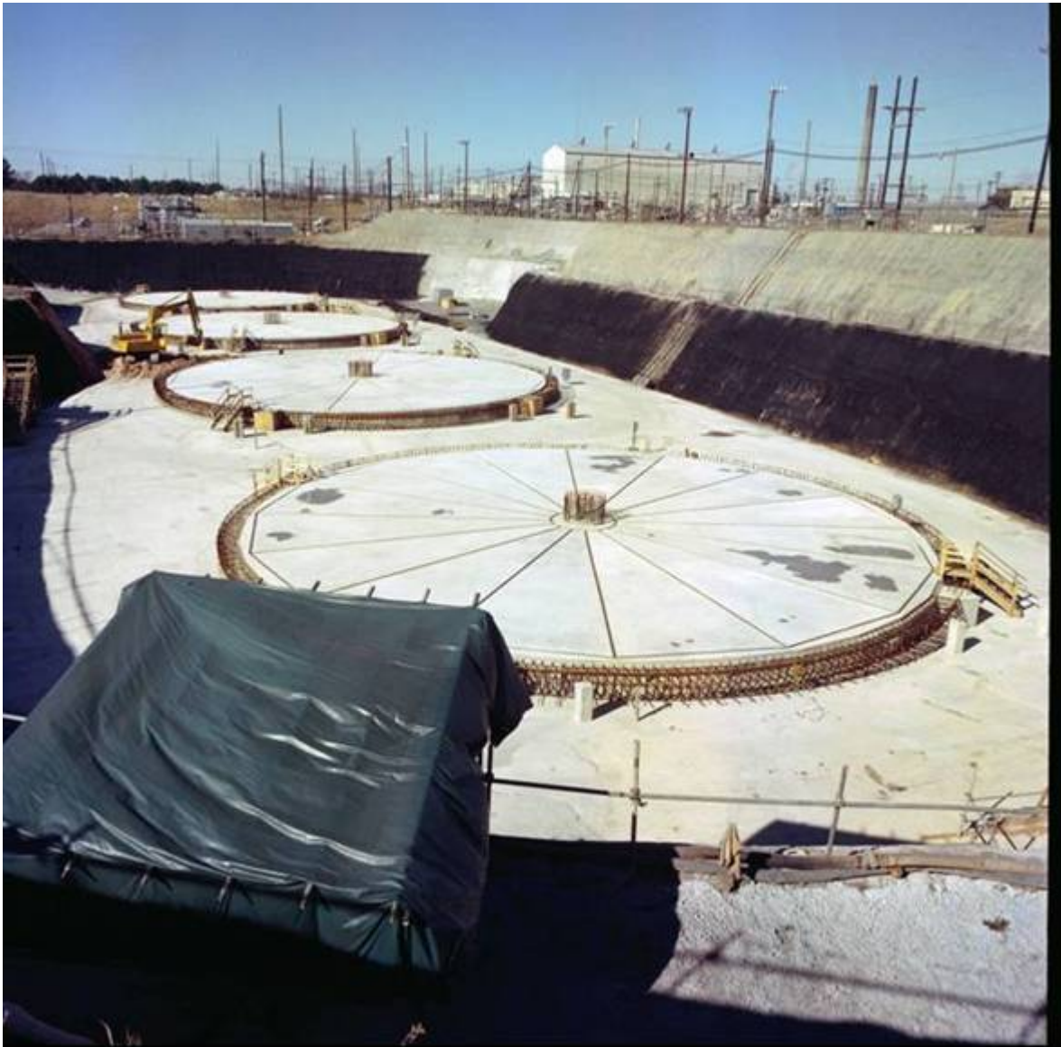
Figure 3.2-17: Tanks 25 through 28 Completed Basemat
