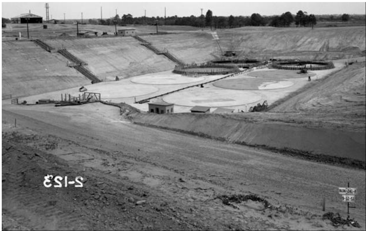
Figure 3.2-4: Tanks 1 through 8 Basemat Construction
