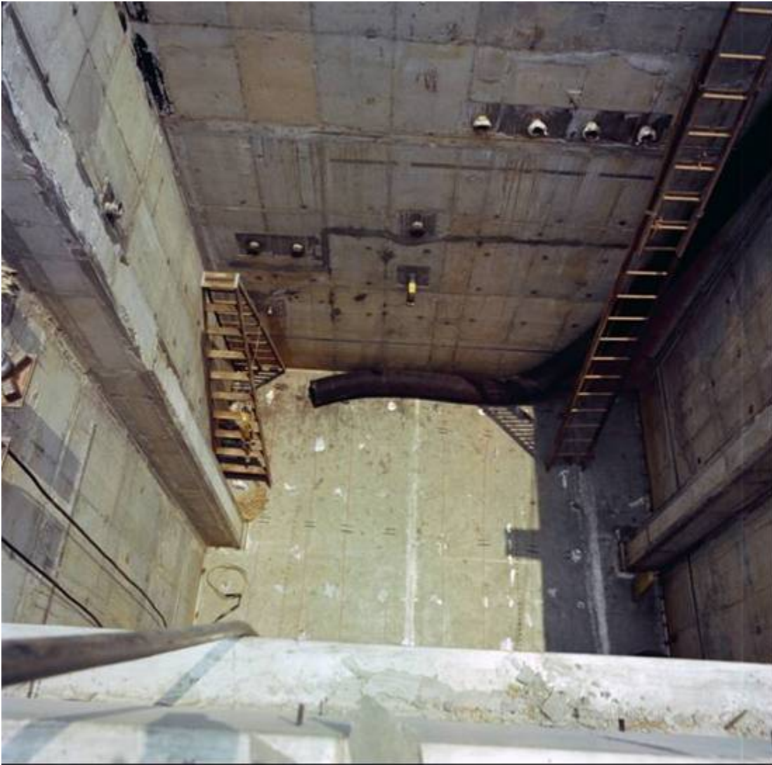
Figure 3.2-44: FPP-2 Concrete Vault During Construction (View 2)
