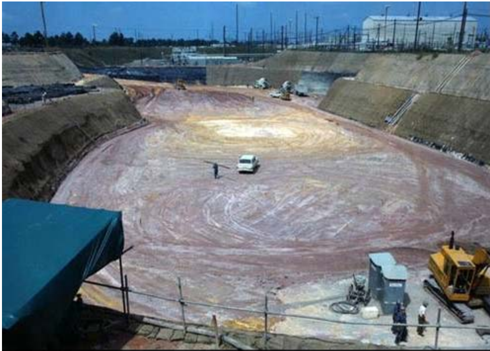
Figure 3.2-16: Early Construction of a Type III/IIIA Tank Basemat
