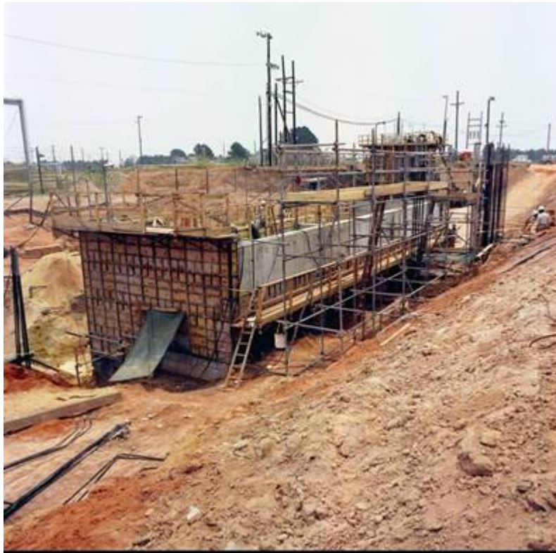
Figure 3.2-42: FDB-4, FPP-2 and FPP-3 During Construction
