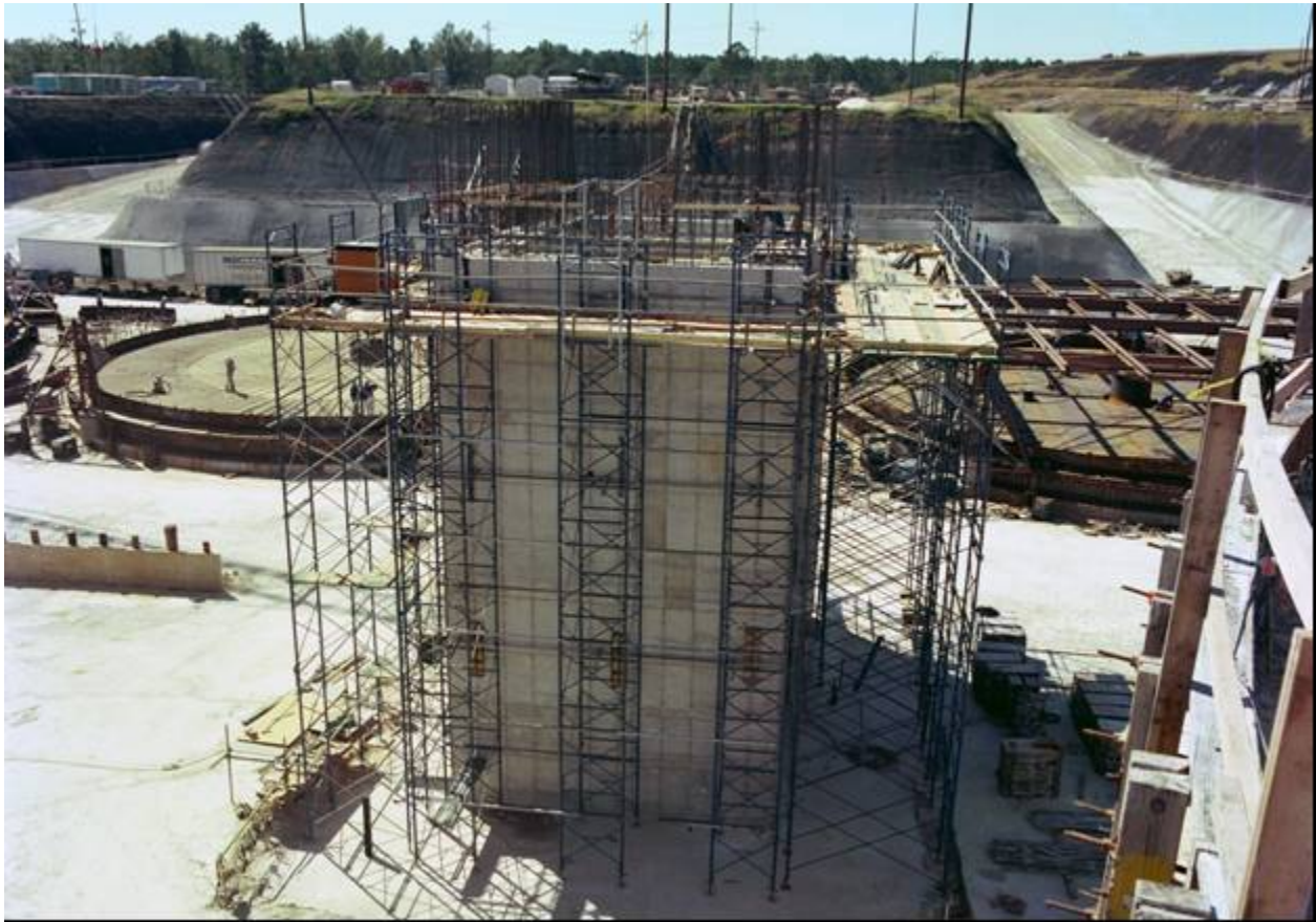
Figure 3.2-53: 242-16F Evaporator Cell Later Construction Phase
