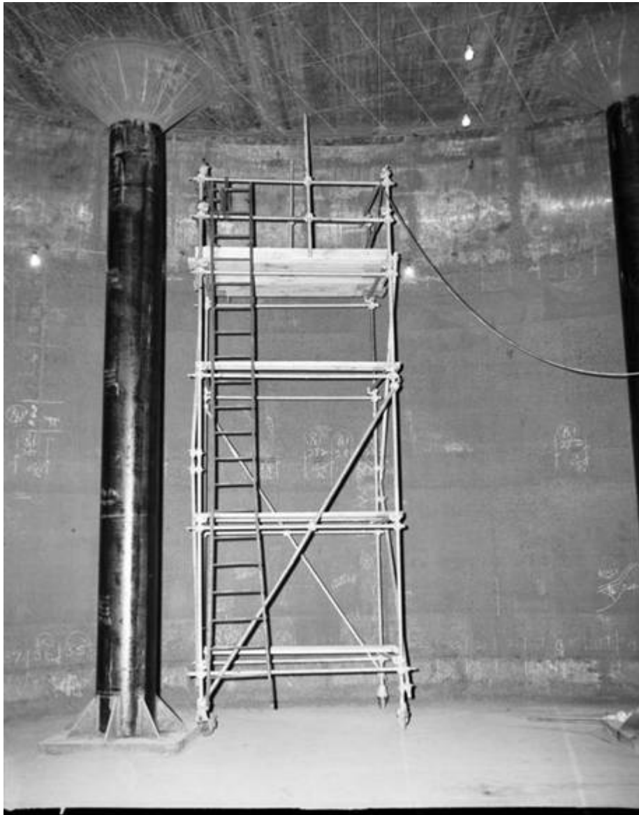
Figure 3.2-10: Support Column During Construction
