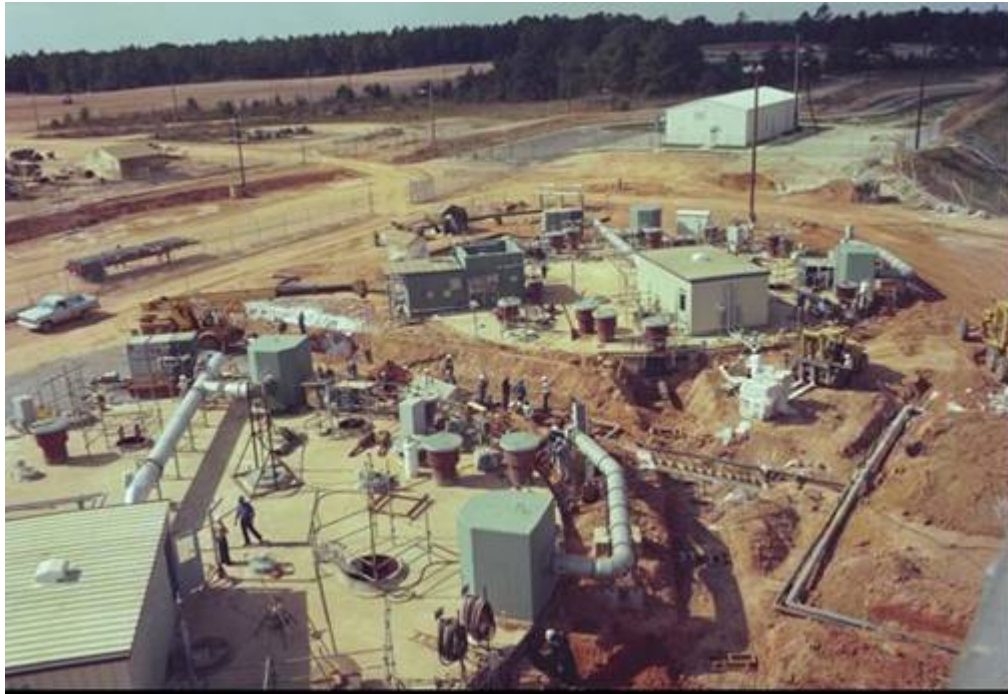
Figure 3.2-36: Transfer Line Construction Near Tanks 46 and 47
