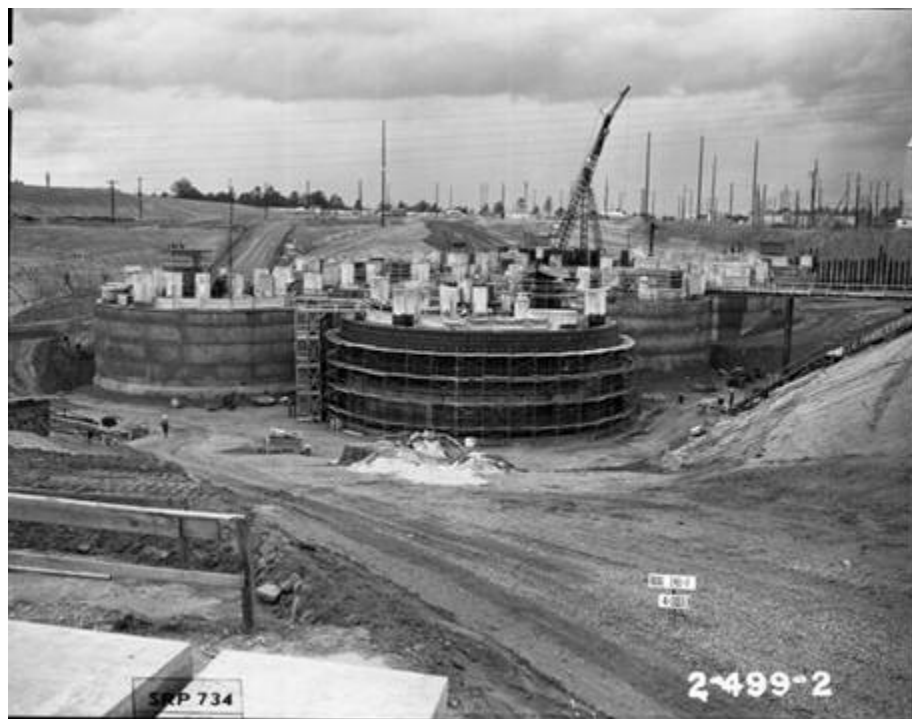
Figure 3.2-9: Tanks 1 through 8 Riser Construction
