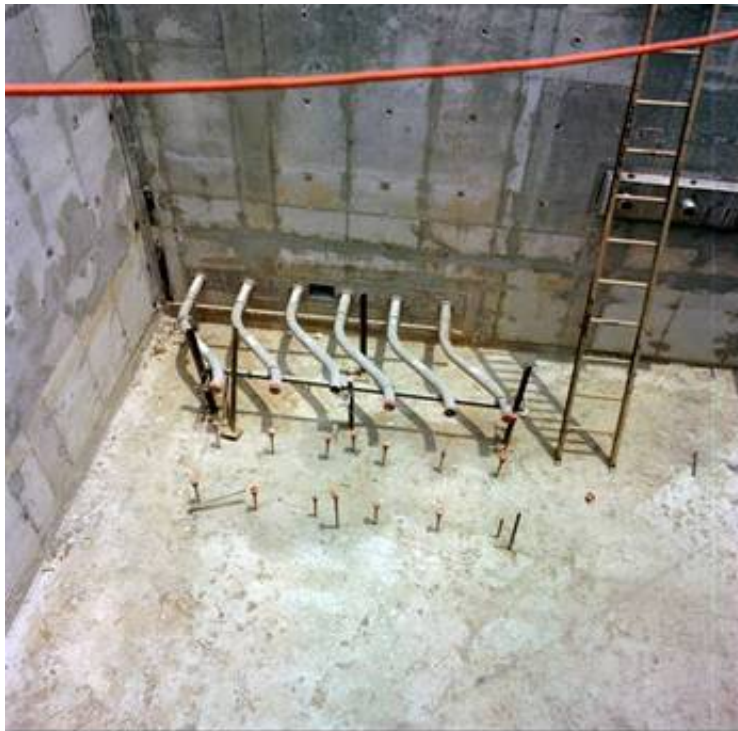
Figure 3.2-55: FDB-4 Concrete Vault During Construction (View 2)
