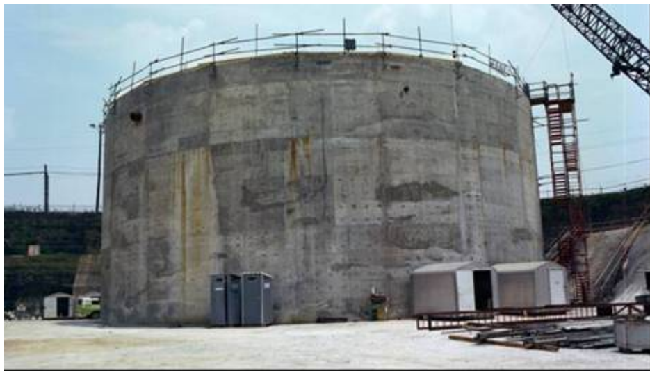
Figure 3.2-25: Final Construction of a Type III/IIIA Tank
