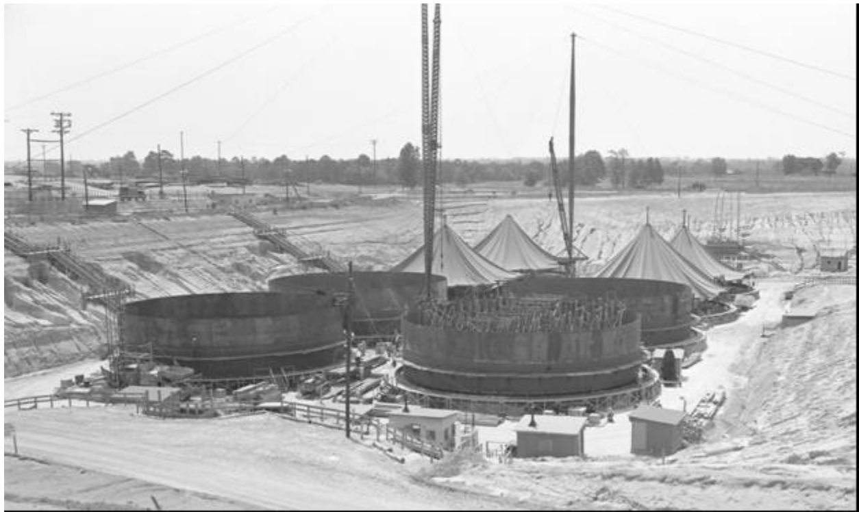
Figure 3.2-5: Tanks 1 through 8 Steel Liner Construction
