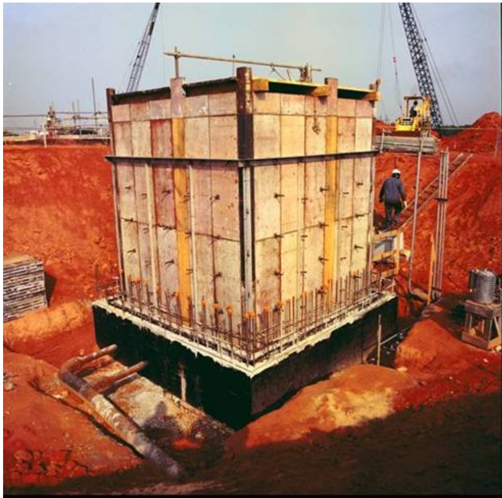
Figure 3.2-56: Diversion Box Early Construction Phase
