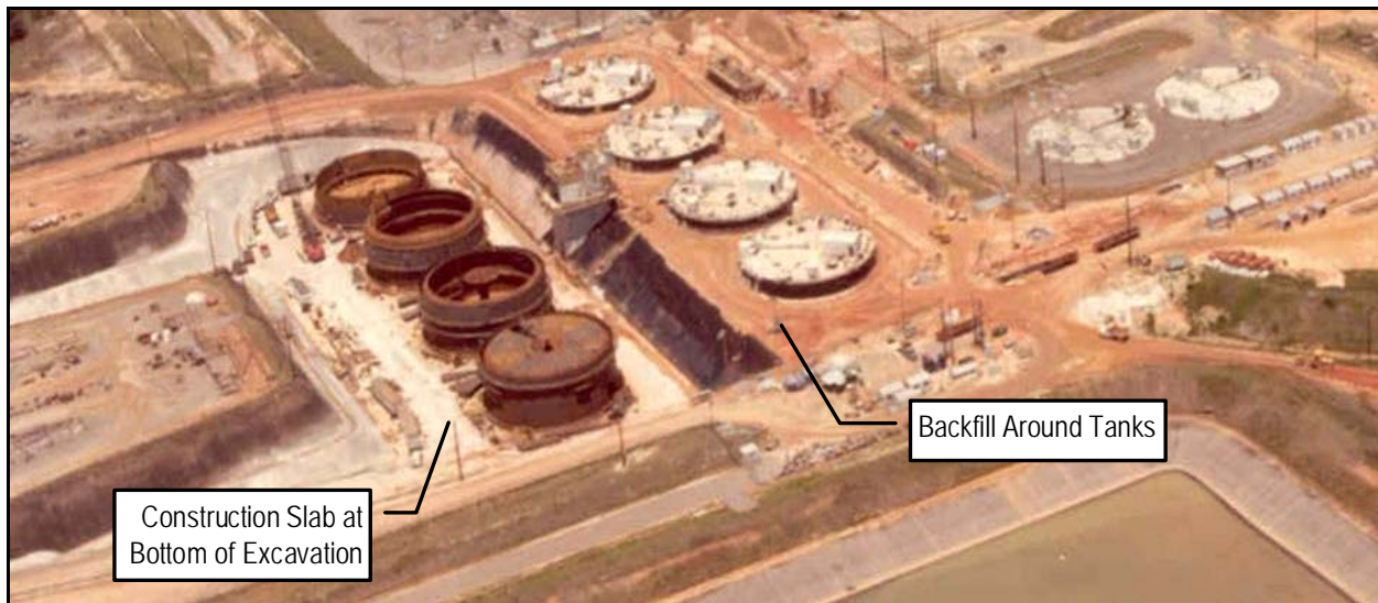
Figure 4.2-18: Type III Tanks under Construction at FTF
