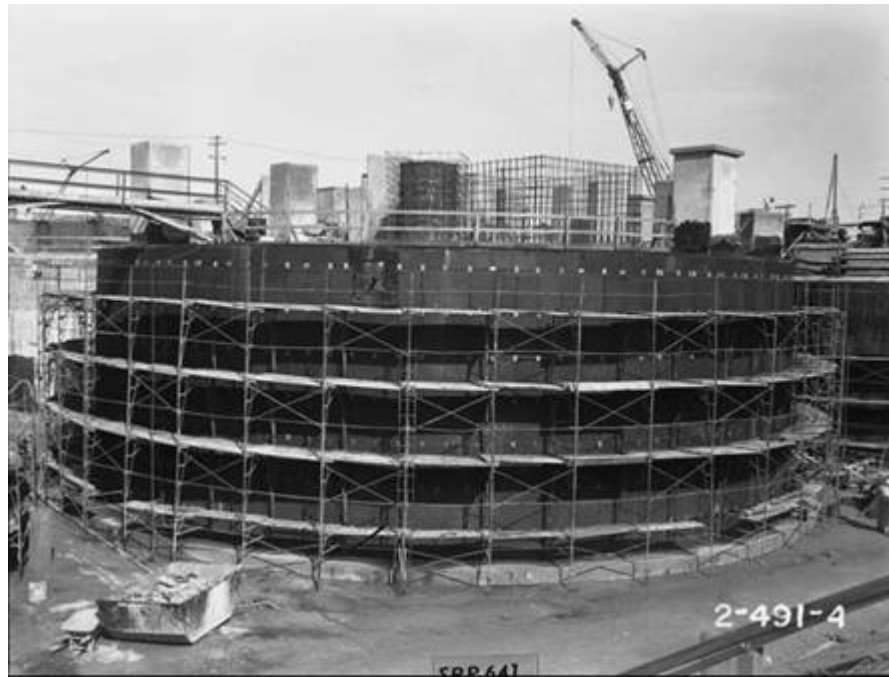
Figure 3.2-9: Tanks 1 through 8 Riser Construction
