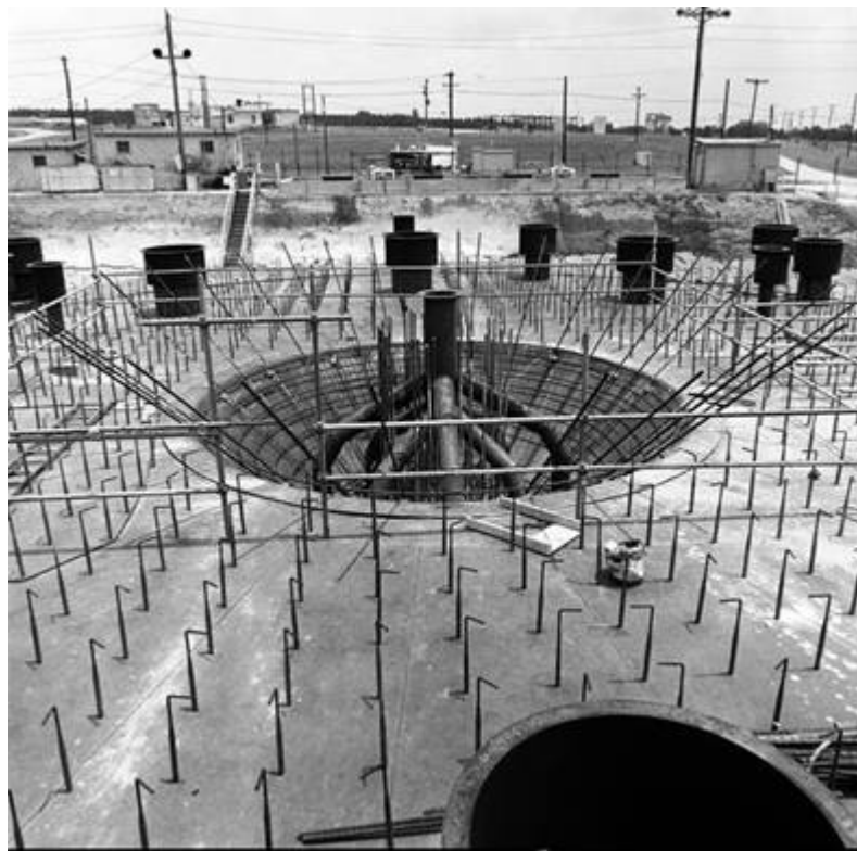
Figure 3.2-23: Tank Top Preparation for Concrete Pour
