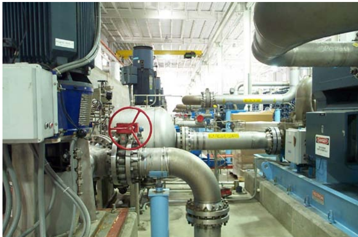
An interior view of Tampa Bay Water's seawater desalination facility on Tampa Bay.
