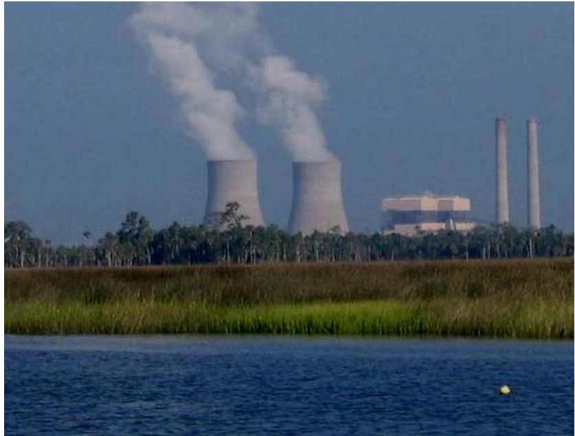
Co-location of a seawater desalination facility with the Crystal River Power Station is a potential water supply option for the Planning Region that could be viable over the long term when available groundwater supplies have been fully developed.
