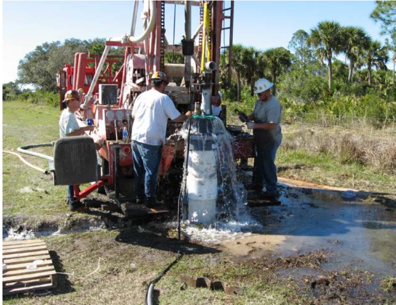
The construction of a groundwater production well. A large portion of 2030 water supply demand in the Planning Region is projected to be met with fresh groundwater.
