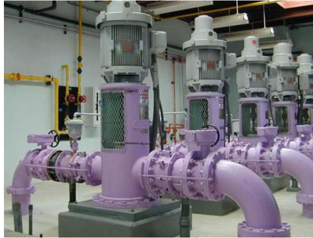
The District strongly promotes the use of reclaimed water including providing matching funds to utilities to develop infrastructure such as this reclaimed water pump station.
