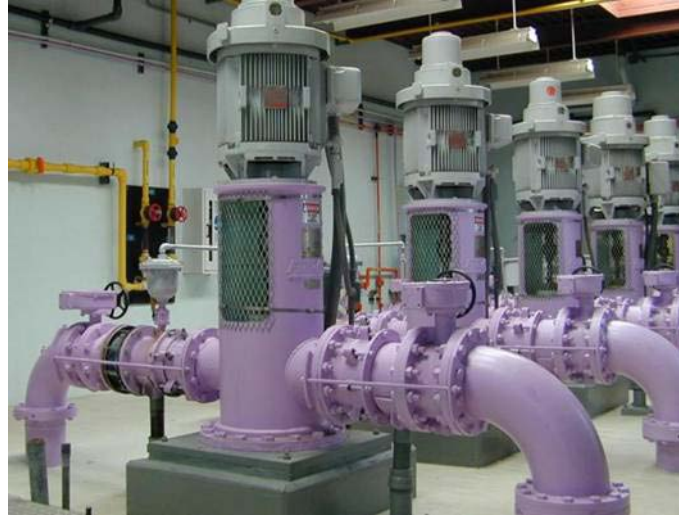
The District has provided hundreds of millions of dollars in matching funds to local governments to develop water supply infrastructure like this reclaimed water pump station.
