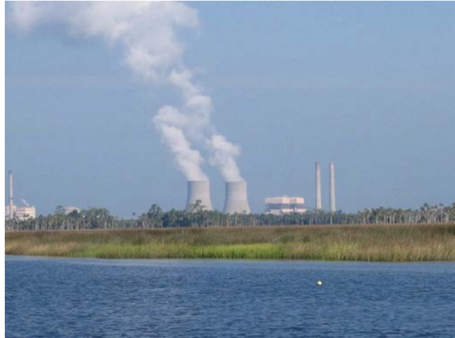
Progress Energy's Crystal River power station uses billions of gallons of saltwater each day from the Gulf of Mexico for cooling purposes. The facility also uses much smaller quantities of fresh groundwater that could be reduced or replaced with reclaimed water from nearby communities.
