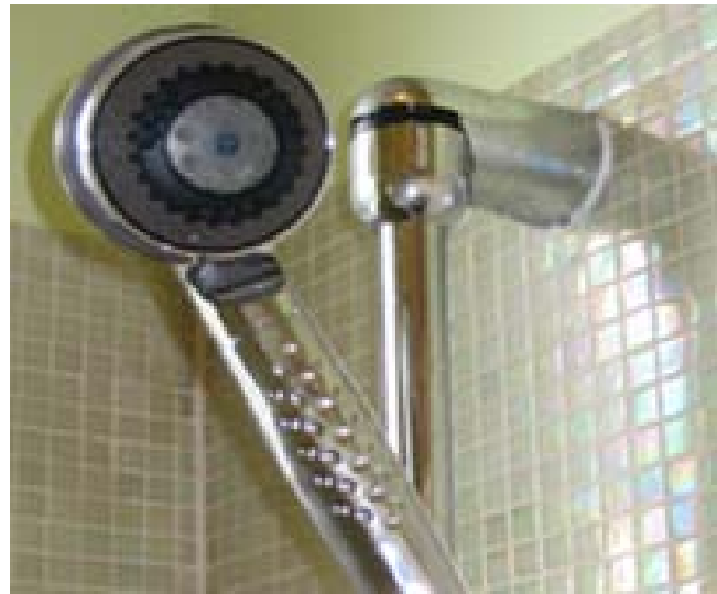
The District assists utilities with the development of incentive programs that encourage their customers to install water saving fixtures such as low-flow shower heads.
