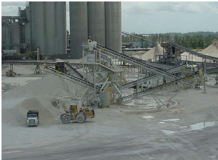
Numerous limerock mines are located in the Planning Region. The demand for water for mining and other industrial uses in the Planning Region is projected to decrease during the planning period.
