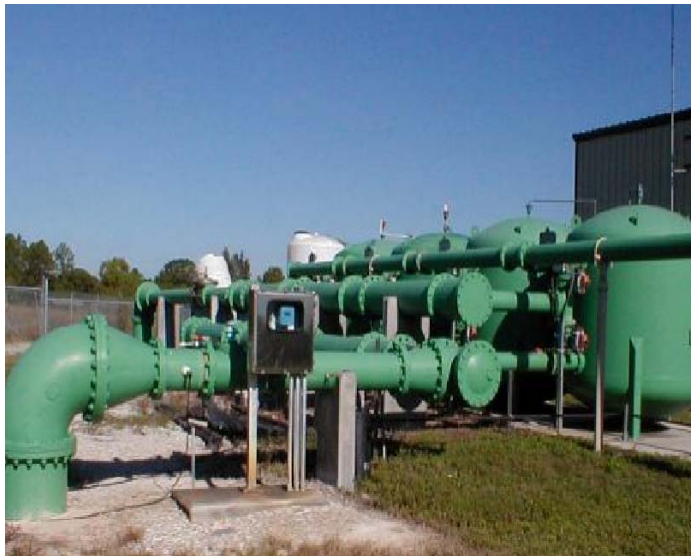
The pretreatment component of a brackish groundwater reverse osmosis treatment facility. Such a facility could someday be developed in the Planning Region to desalinate water from the Lower Floridan aquifer.
