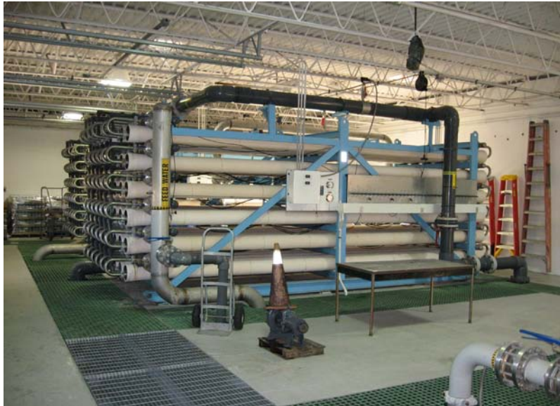
Reverse osmosis membranes in a brackish groundwater treatment facility.
