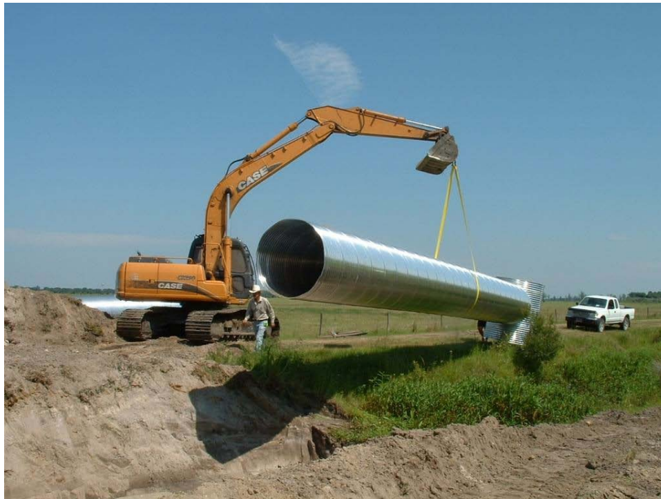
Installation of a culvert for a tailwater recovery project in the Southern Planning Region that will recover and reuse excess irrigation water. The District will provide funding for similar projects in the Northern Planning Region.
