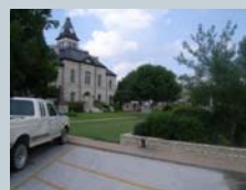
Somervell County Court House Source: PNNL
