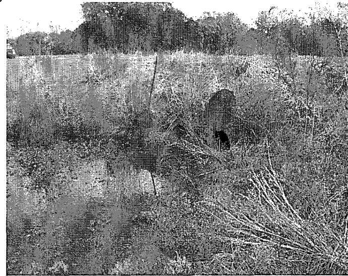
Culvert in Activity Area
