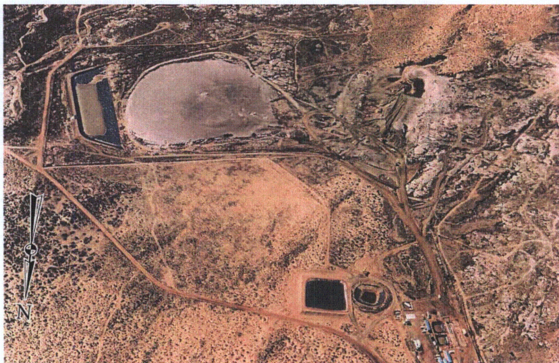
Figure 2-5. Contaminated Excavation and Haul from the Heap-Leach Area Prior to New Tailings Pile and Evaporation Pond Excavation (March 1993)
