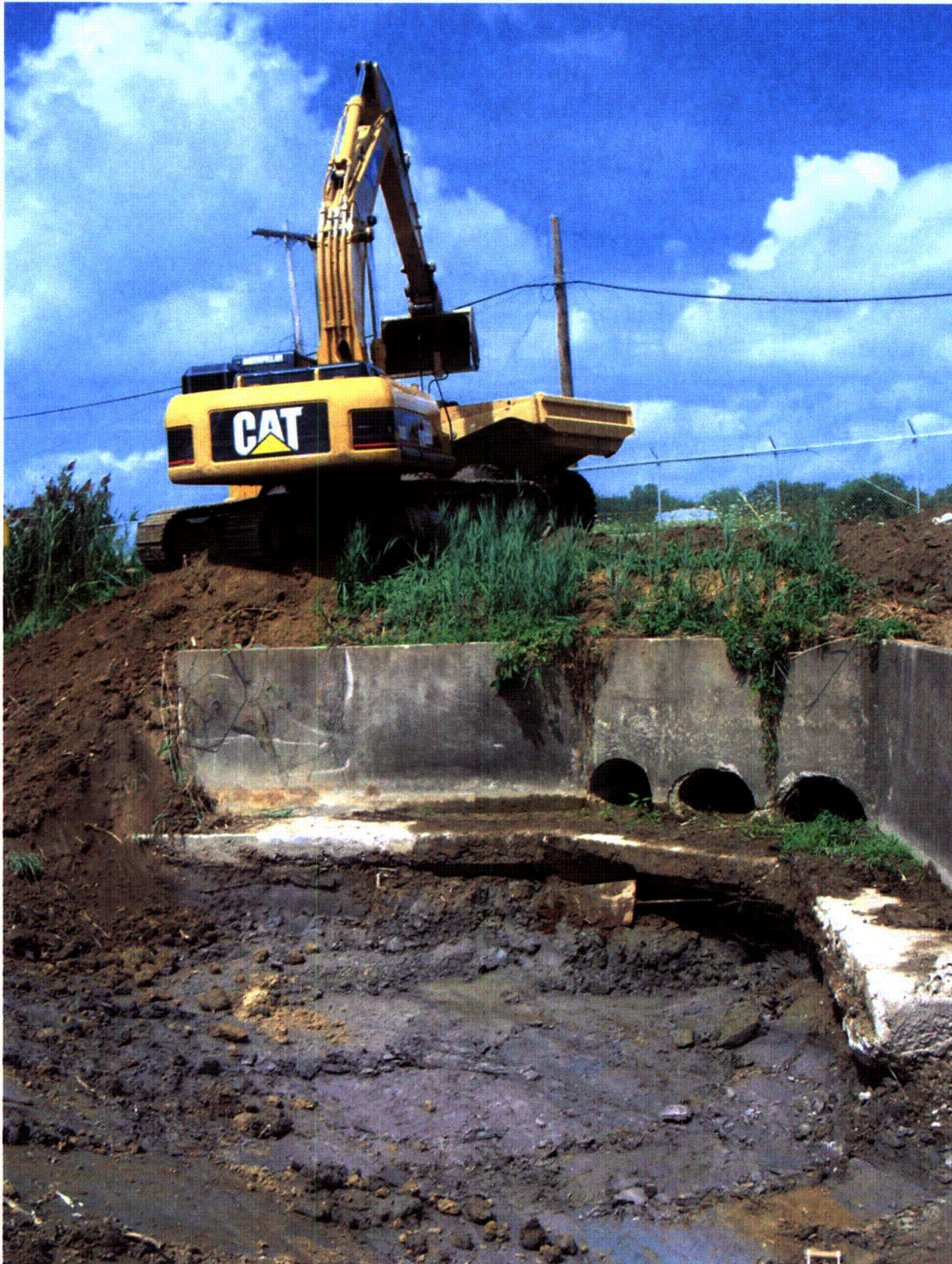
Exhibit 15, Excavation of WEMS Outfall Load-out of Sediment at WEMS Outfall
