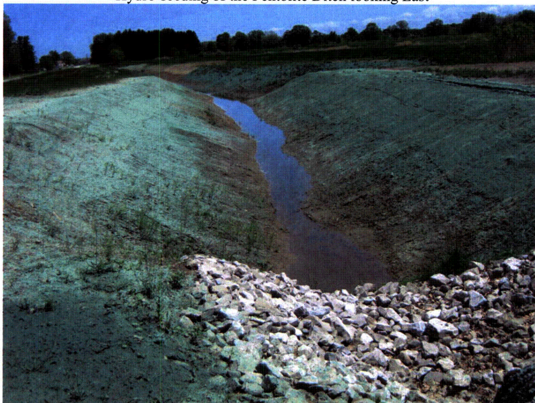
Hydro-seeding of the Pentolite Ditch looking East
