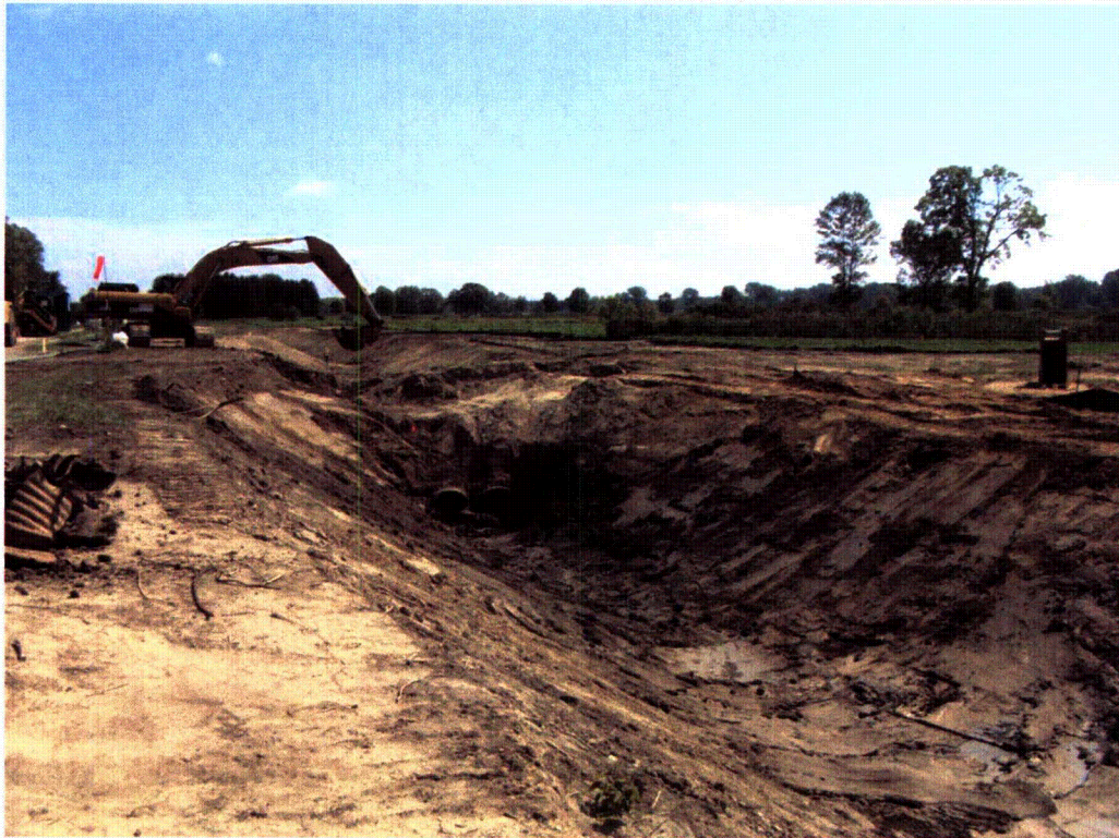
Excavation of Pipe Culverts
