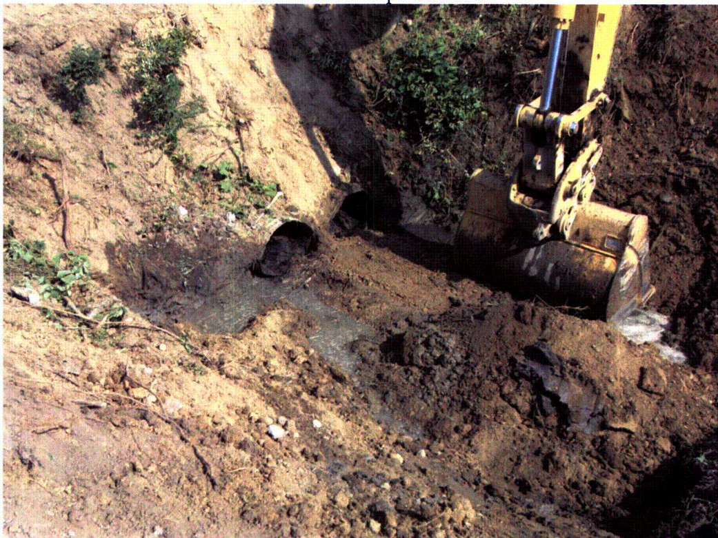
Excavation of Pipe Culverts
