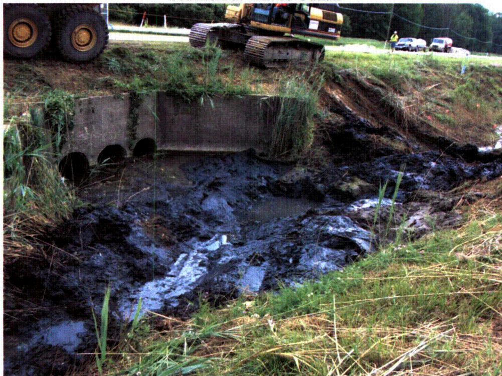
Excavation of the WEMS Outfall
