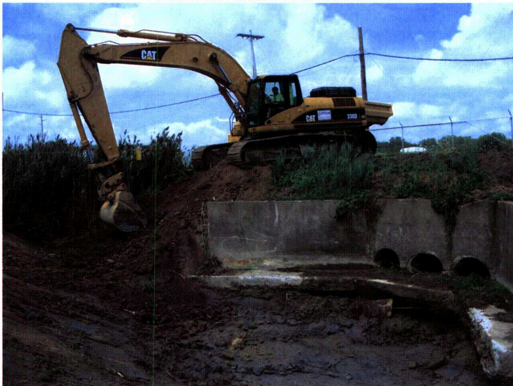
Excavation of the WEMS Outfall
