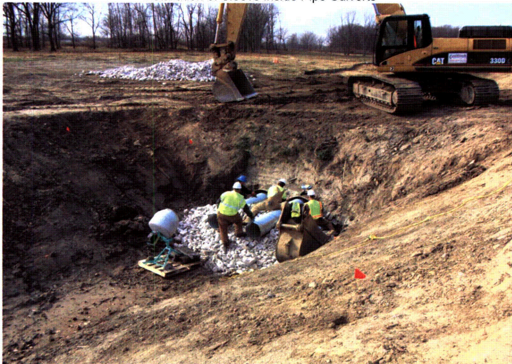
Installed Pipe Sleeves
