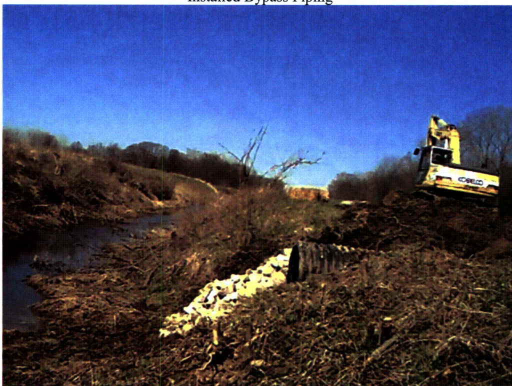
Installed Bypass Piping
