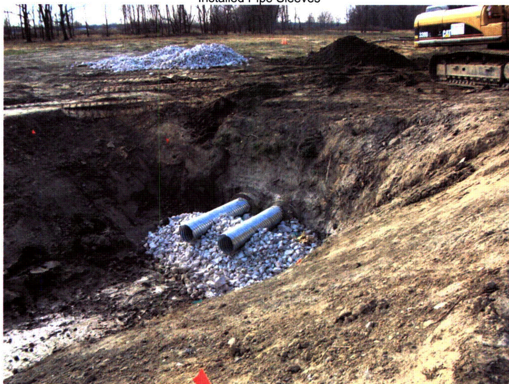
Installed Pipe Sleeves
