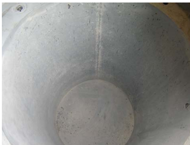
Post Test View of Inner Containment
