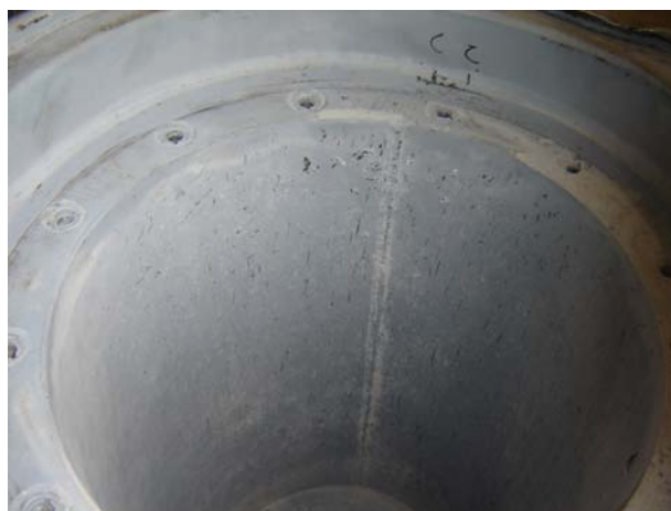
Post Test View of Inner Containment
