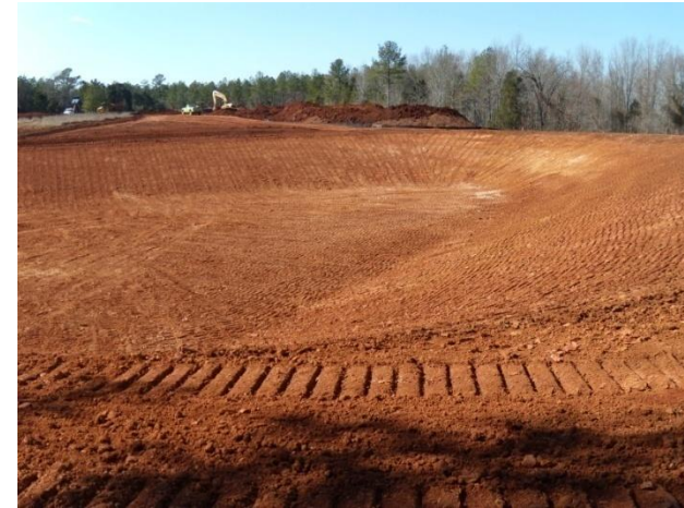
Sediment Pond Excavations
