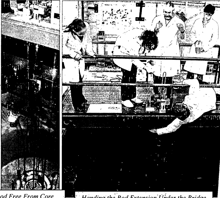
Handling the Rod Extension Under the Bridge
