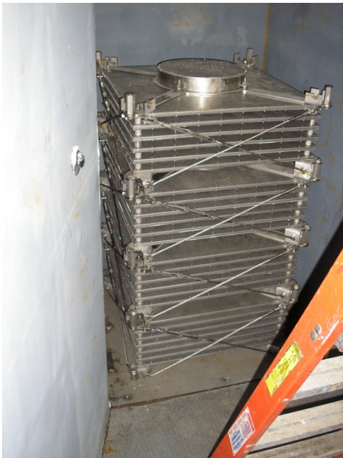
Photo 1-Strainer in Tank
