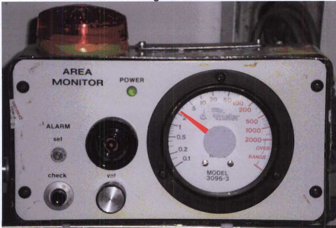
Refuel Platform ARM (AM-2) Indication
