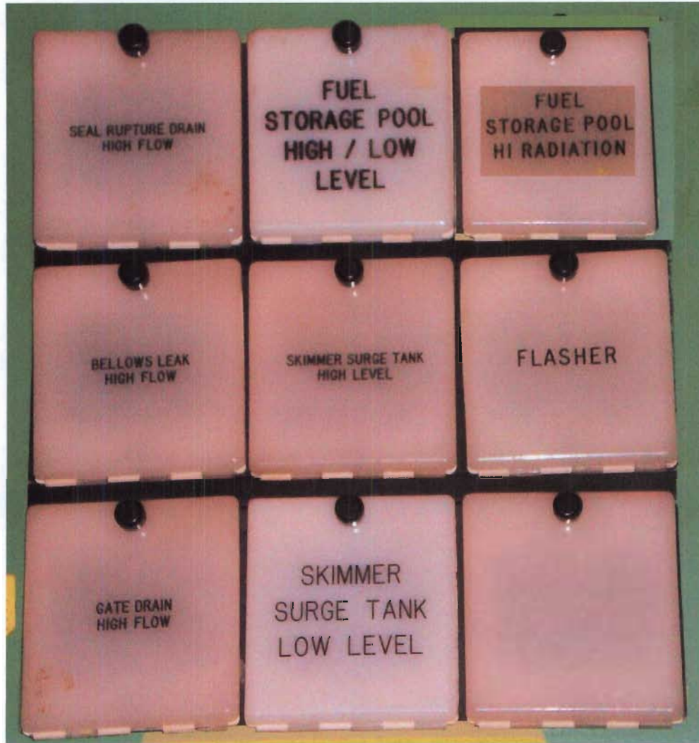
Fuel Pool System Instrument Rack 20C075 Alarms
