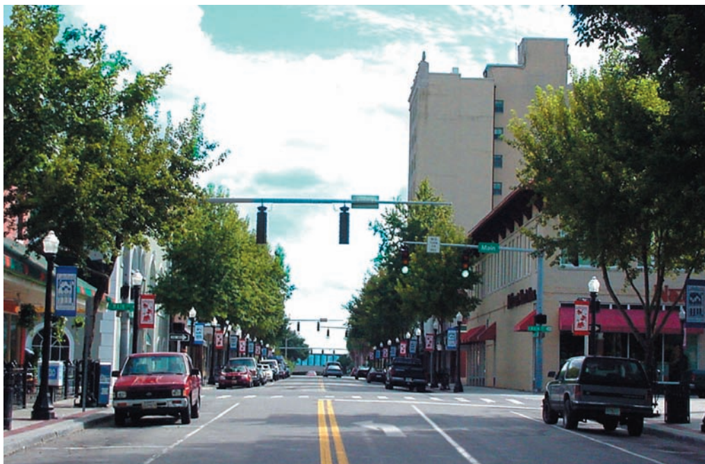
Figure 91. Three-lane street configuration with on-street parking, Lakeland
