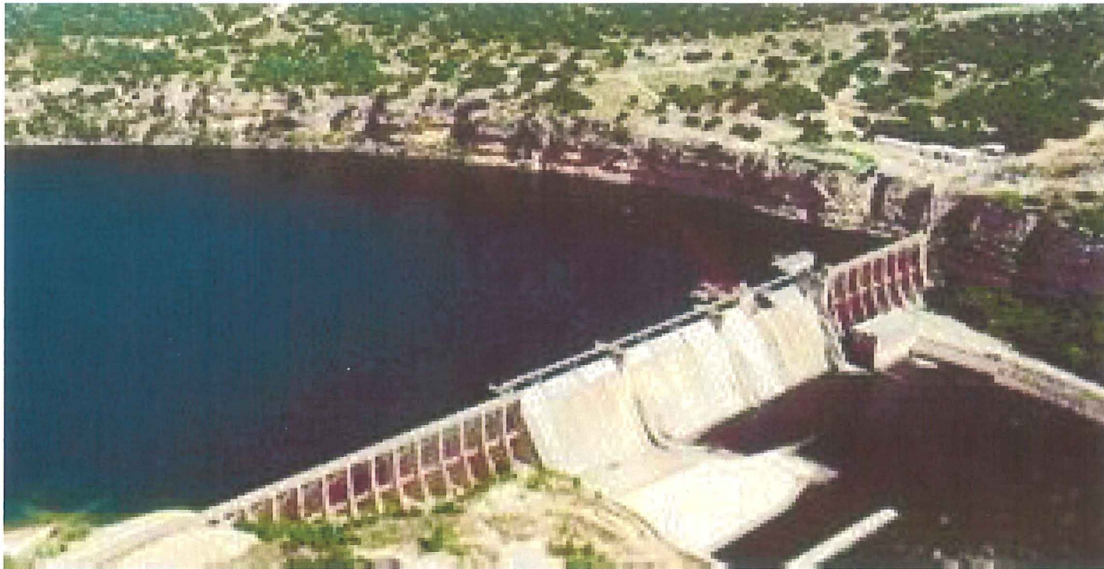
Figure 7-35. Morris Sheppard Dam (Reference 5)
