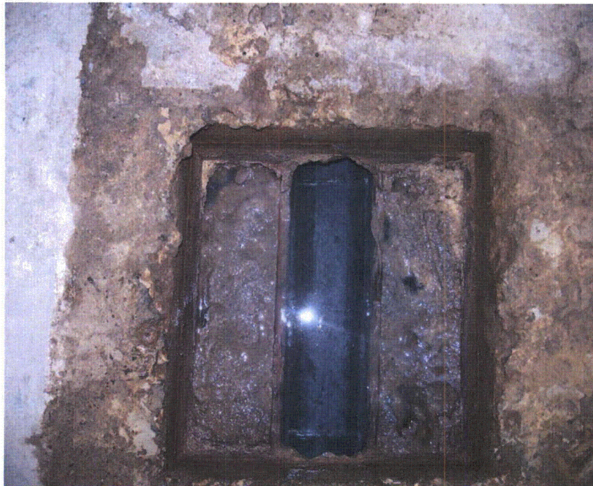
Floor Drain Access near Vault Center Showing Clay Tile Drain Piping (Survey Unit HR-1-5)
