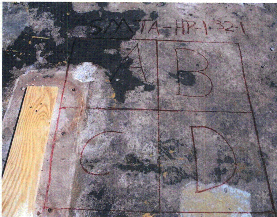
Chipped Concrete and Roof Coating Remnants on Pipe Chase Roof
