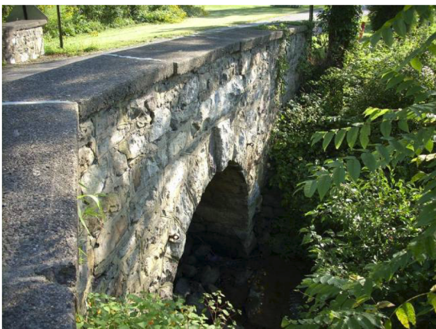
Photograph 7. Lot 4, Stone Arch Bridge (GAI-06), Facing Northeast
