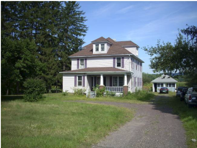
Photograph 14. Lot 96, Section 1, Showing GAI-24 (Abandoned Dwelling and Garage), Facing North
