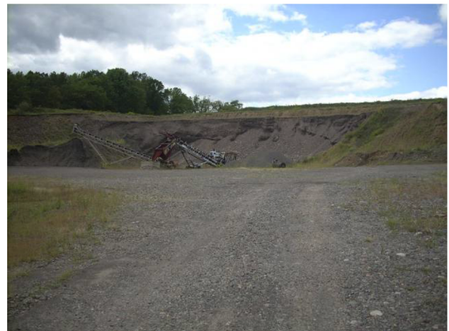
Photograph 17. Lot 100, View of Quarry at Eastern Edge of Section 2, Facing Southwest
