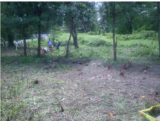
Photograph 18. Site 7, Locus 2, Showing Shovel Testing in Area of Structure 2 (House Foundation), Facing West
